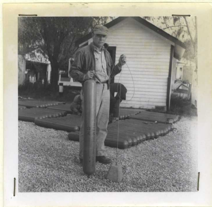
Maintenance man Snider with floating buoys and anchor assembly used to mark boundaries of refuge units at Lake St. Clair.
