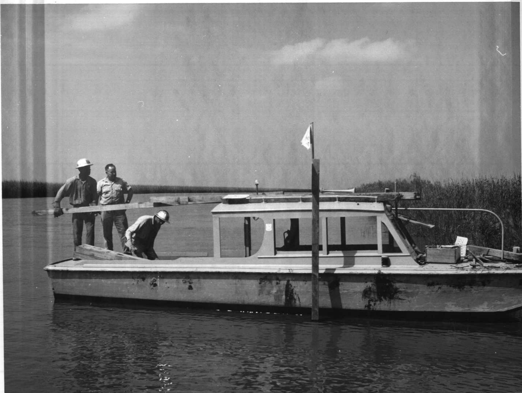
4 Boundary and interior posting operations. Seventeen navigable passes and bayous constituting 160 miles must be adequately posted. All operations must be by boat. Fourteen foot treated 4x4 posts are necessary for stability in this deltaic silt and against storm tides.
