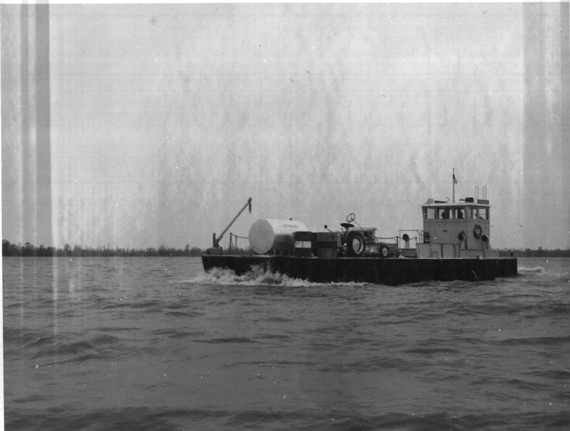
3 An unusual but prime piece of equipment at Delta. A military landing craft converted to a flush-deck cargo vessel. All supplies, equipment and material must be moved over 8 miles of water from the Port of Venice, La. to the island headquarters.
