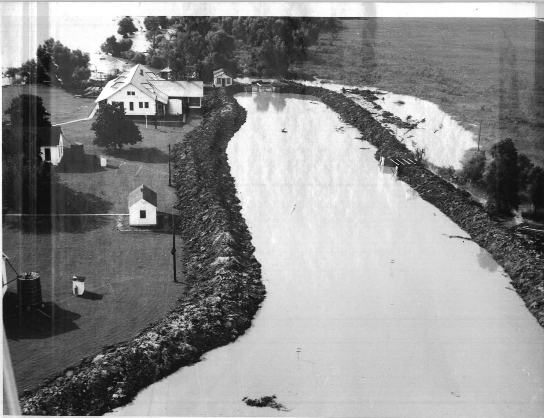
Northern end of headquarters and part of the 200,000 cubic yards of fill pumped in to raise the elevation of the headquarters site. Fill was extended to this end to provide additional runway space for the landing strip.
