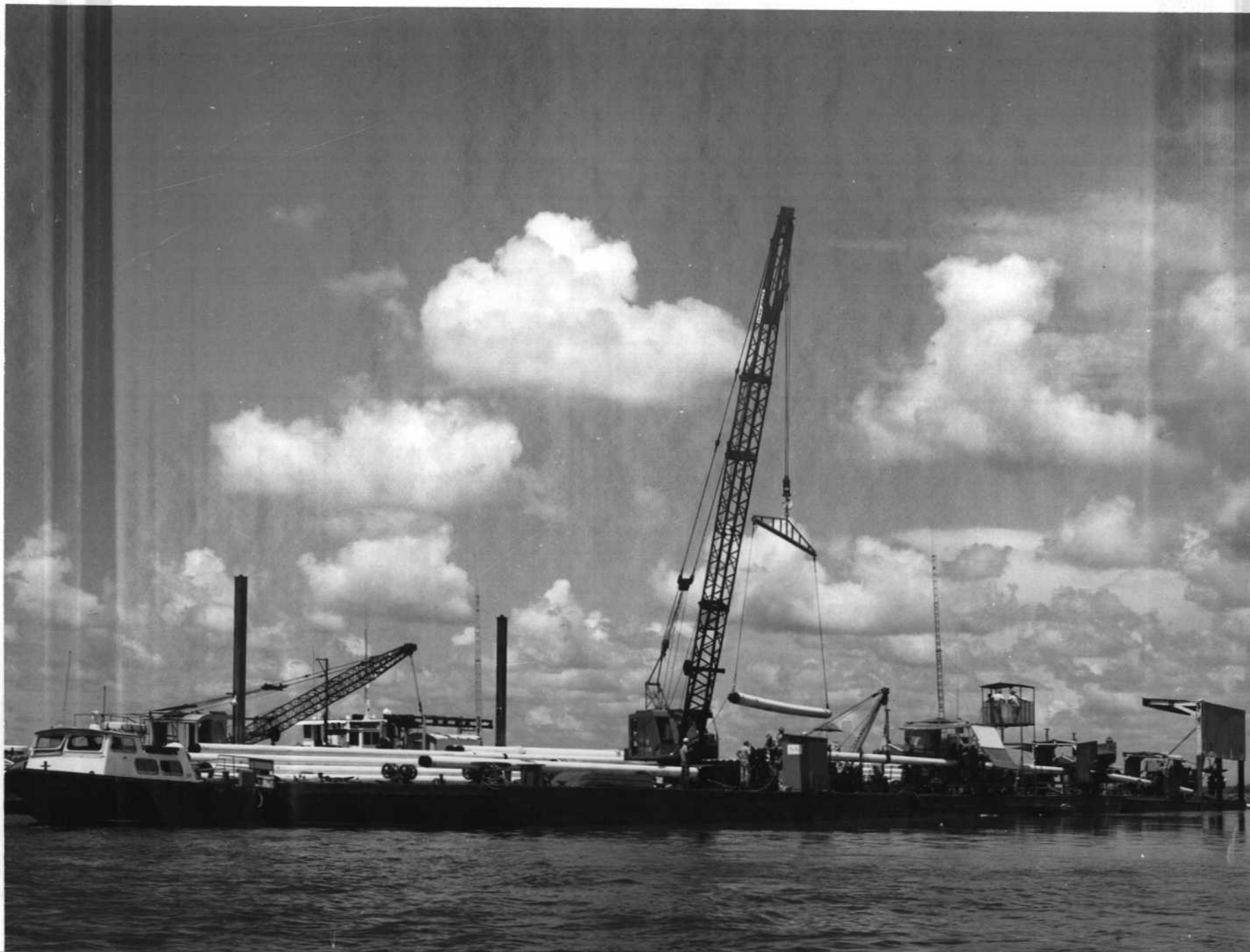
Pipe-laying operations across refuge lands. The old days of the wide, deep pipeline canals are over. This 400 ft. lay barge is capable of automatically welding, ex-raying and pushing four miles of 14" pipe in a very narrow slit trench without moving location. Marsh disturbance is reduced to a minimum.
