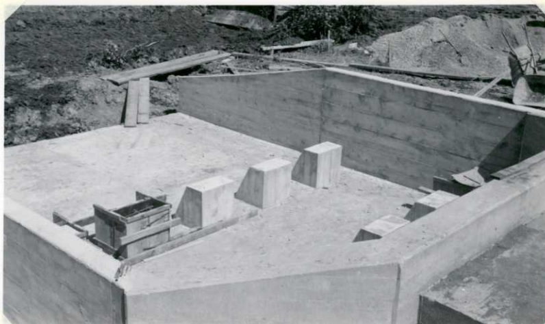
Photograph # 9. Another view of addition to water control structure completed with exception of two baffle blocks. (6-10-52)
