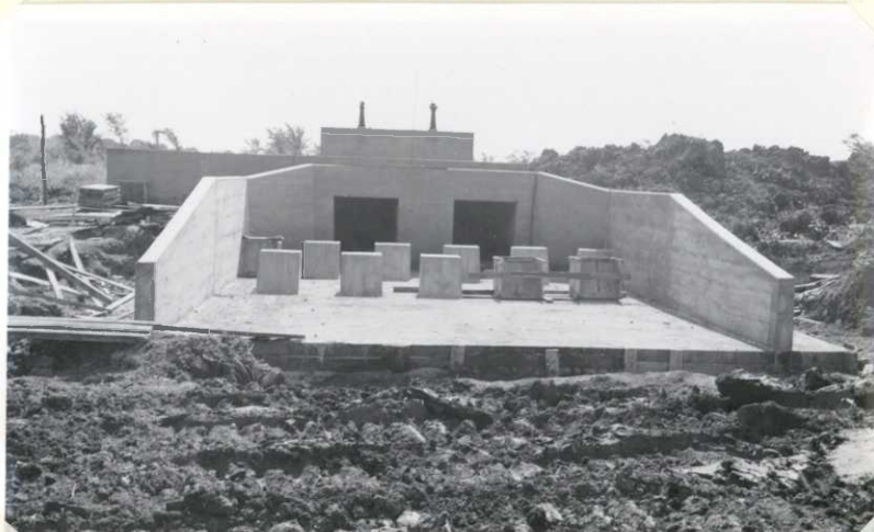
Photograph # 8. Addition to water control structure completed with exception of pouring two baffle blocks. (6-10-52)
