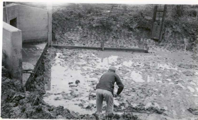
Photograph No. 6. Addition to water control structure. Getting ready to drive piling at west end of Levee # 2 water control structure. (5-16-52)
