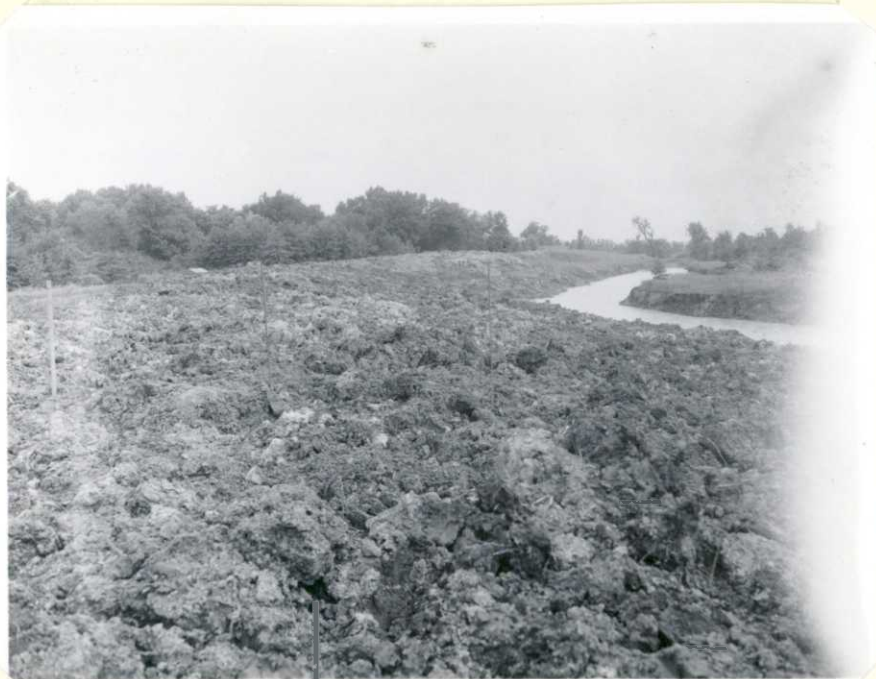
Photograph # 4. Looking north over section of Levee # 2 completed. Note water control structure at arrow. (Exp # 11 - 8-31-52)
