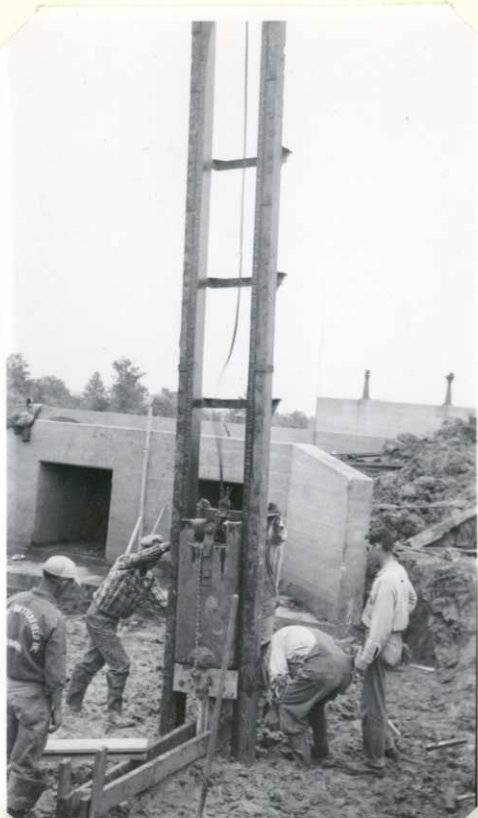
Photograph # 7. Addition to water control structure. Driving piling west side of water control structure Levee # 2. (5-6-52)
