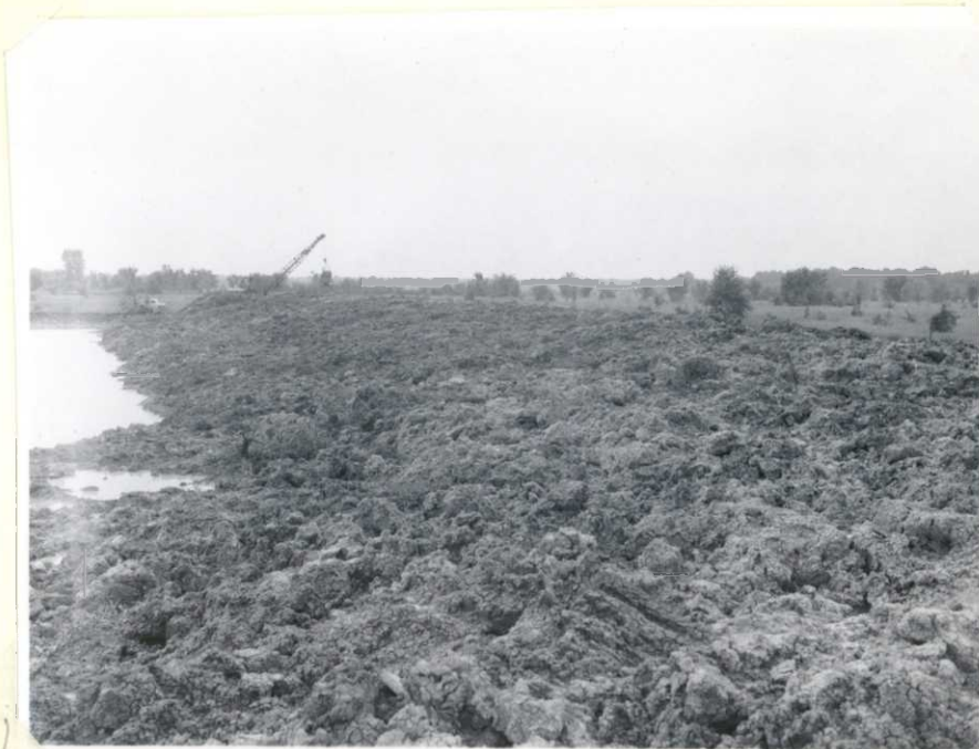
Looking south from water control structure over Levee No. 2 recently thrown up with Model 6 Northwest drag-line. (Exp. # 12 - 8-31-52) Photograph # 5
