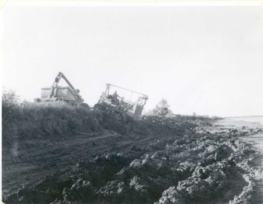
Photograph # 11. D-7, with 6-yard soraper obtained from Necedah refuge, repairing face of Levee # 3 one-half mile south of water control structure. (Exp. 14 - 8-20-52)
