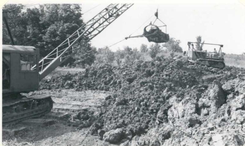
Photograph # 3. Starting Levee # 2 south of Elk Creek. Model 6 Northwest recasting material to form west slope of levee. D-7 tractor with dozer shaping and smothering up. (6-1-52)
