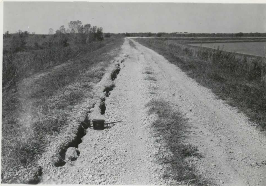
Crack in Levee No. 1. In some places levee shoulder has dropped 1 - 3 feet. (Exp 41 - 10-4-53)
