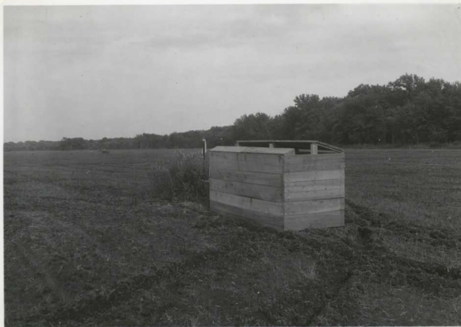
Front view of pit in wheat field before being "dug in". Dimensions! 4' x 4' x 8'. Accomodates four hunters. Constructed of green cypress. Front top is hinged to fold forward. (Exposure No. 141, 9-10-55)
