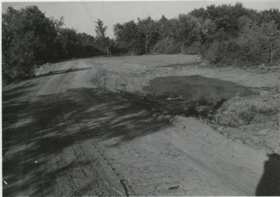
Typical section of old farm levee cleared and graded for access road. Note parking area upper center. (Exposure No. 139, 9-10-55)
