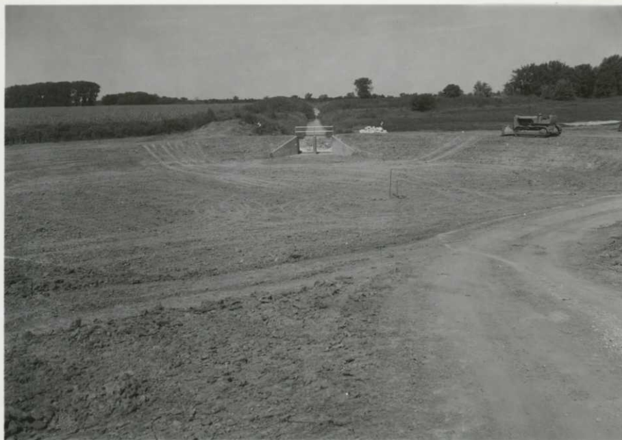
Swan Lake diversion structure nearing completion. Distribution basin in foreground. (Exposure No. 137, 9-10-55)
