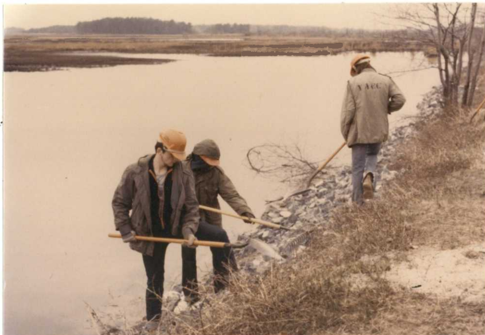
80-C-8 YACC placing riprap. Photo by K. Kammeyer
