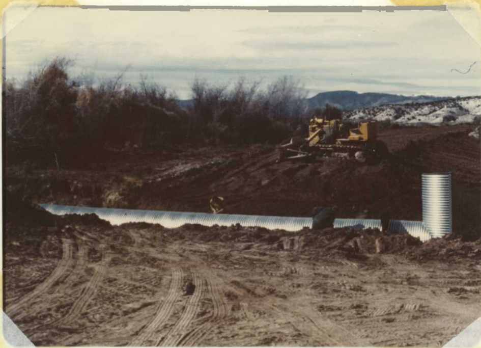
Putting in drop gate and CMP for Beaver Creek Crossing, a BLHP project. March '78. J.C.
