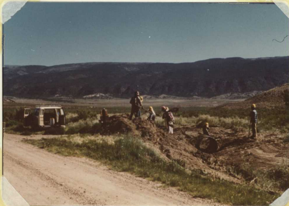
A YCC crew replacing a wooden bridge with a culvert in the Hoy delivery ditch. 7/14, J. Creasy
