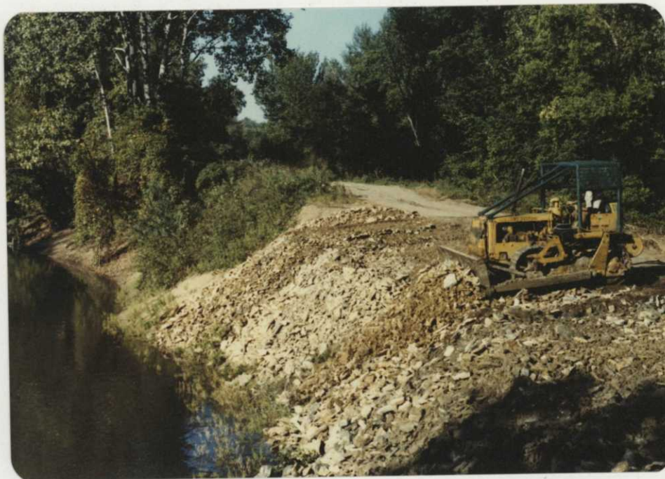
REHAB of the south dike required gravelling 0.7 miles of trail in order to place 290 tons of rip rap at the Quiver Creek Weir.
