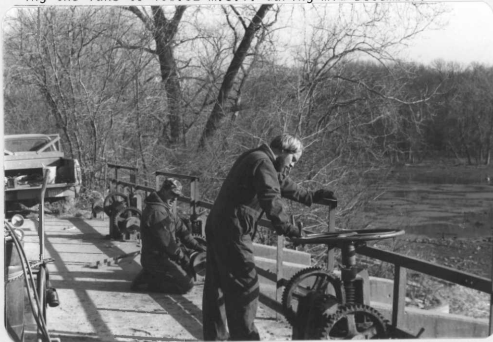
Radial gates became operative after replacement of cables.
