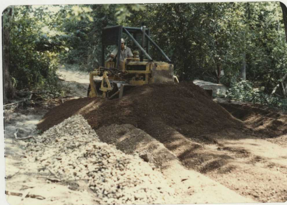
Repairs to north dike by spreading 290 tons of CA-6 and over size rock.
