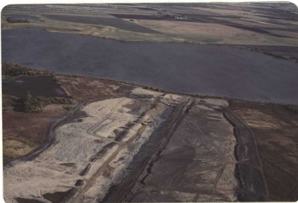
Channel "A" water control structure below Dry Lake. Note unfinished segment of channel between structure and the lake--the infamous "200 ft. plug".
