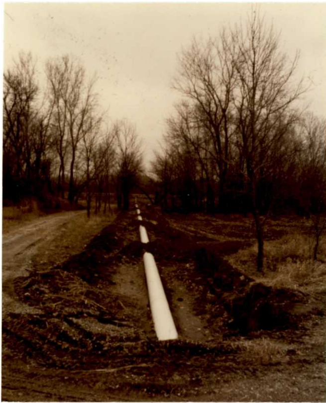
A 375-foot PVC pipeline was laid to pump water from the Missouri River to the Nebraska waterfowl hunting area. Clawson 11/80
