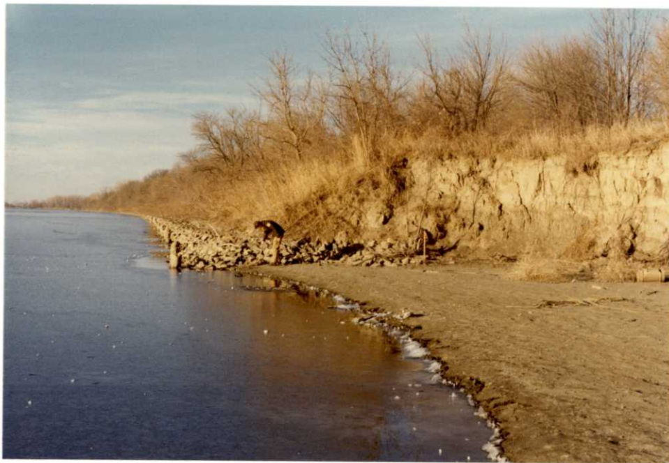
The above photo gives a good comparison between protected (riprapped) and unprotected DeSoto Lake shoreline. Jave 12/80
