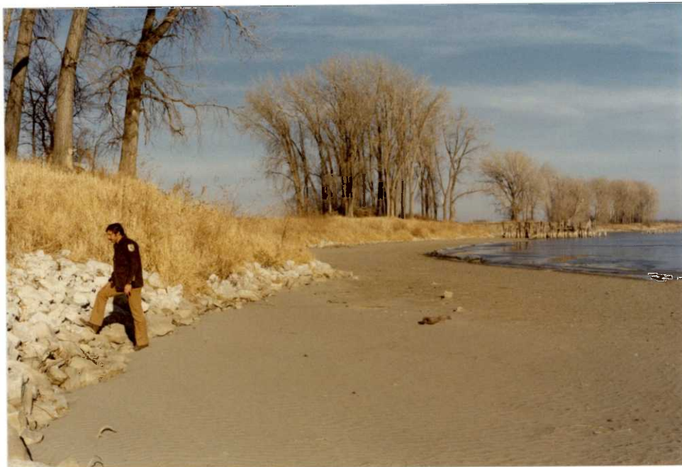
The 1,800 feet of sloping and rip-rapping north of the visitor center healed over fairly well by winter drawdown. Knauer 12/80
