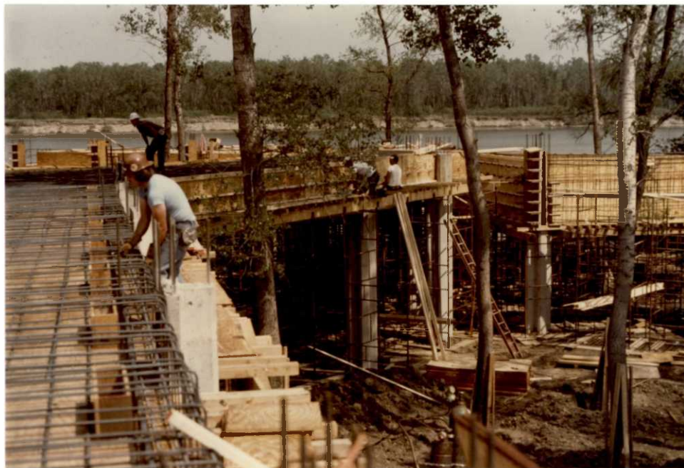
Over 3,600 cubic yards of concrete were poured to form the visitor center's structural shell. Montgomery 5/80
