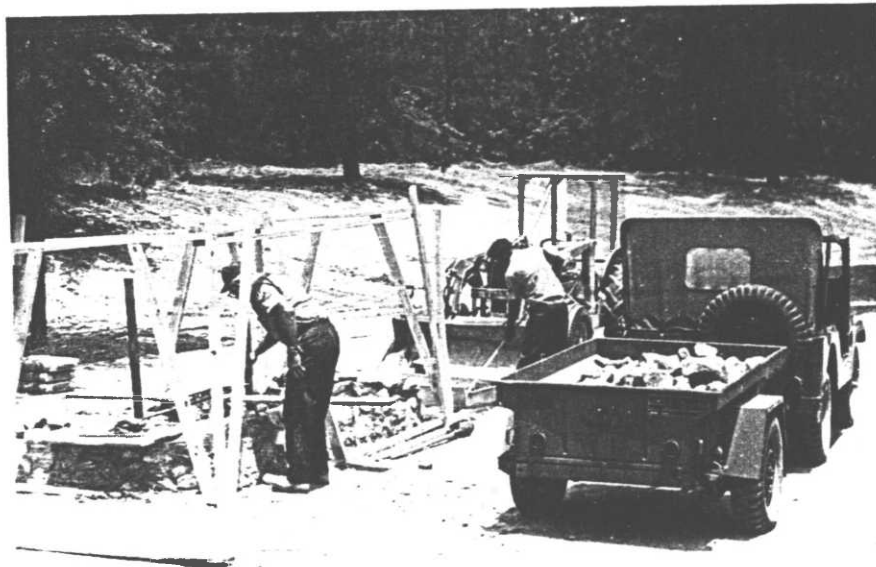
Building sign base from excess rip-rap.
