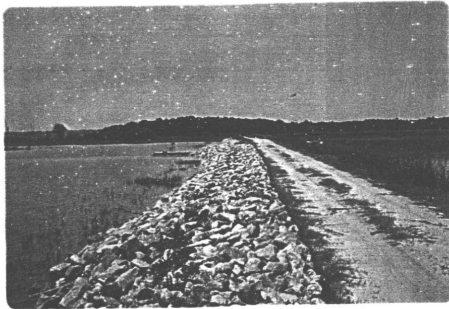
Finished job with hand placed row-line.
