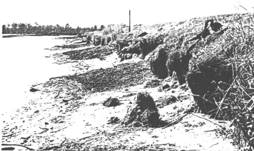
Effects of wind sweep - South Houston. When dike was built it had a 4:1 slope.
