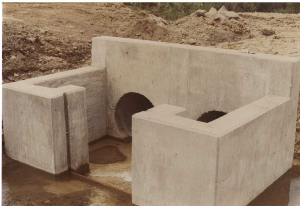
Water control structure box for new headquarters entrance road pool.
