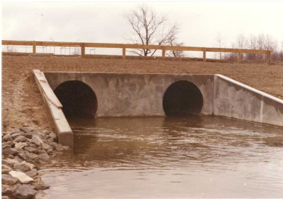
Looking north at new six foot culvert pipes and discharge box for Pool 4 on Township Road 473.
