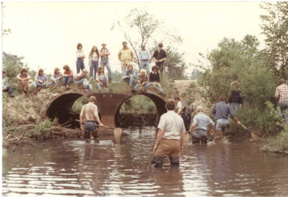
Looking north at railroad tank car culvert pipes installed by township supervisors many years ago to pass Lake Creek through Township Road 473 at the Pool 4 site. Note beaver dam on upstream side of pipes. YCC's of 1980 were observing fish survey.
