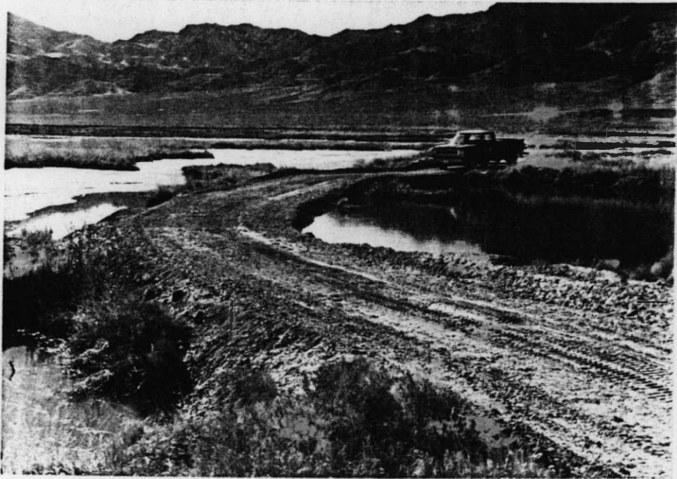
AVOCET UNIT - SAME DIKE Gravel riprap holds water better and is more muskrat resistant.
