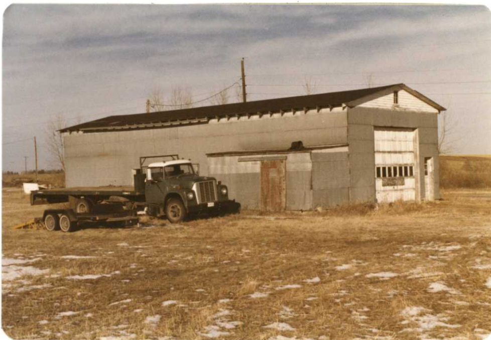
Figure 5. This existing building will be used as a temporary shop and storage building. It is constructed of 2" tongue in groove redwood and is scheduled for remodeling in FY 80 with BLHP funds.
