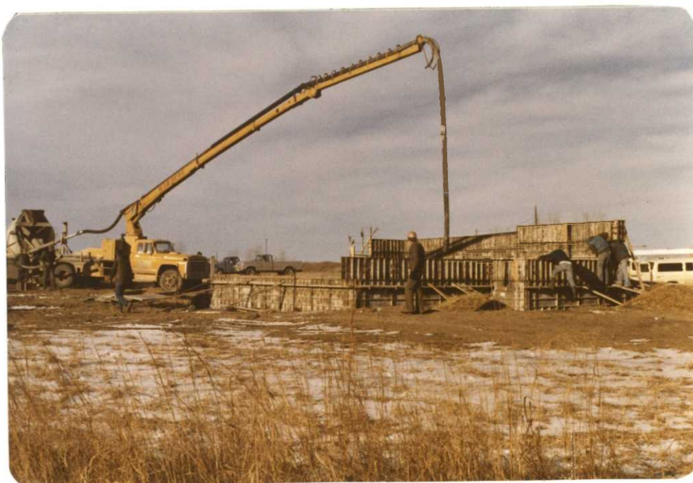
Figure 6. Gilbert inspects the cement pouring for the new office foundation. The temperature on this day, December 18, was 48° F.
