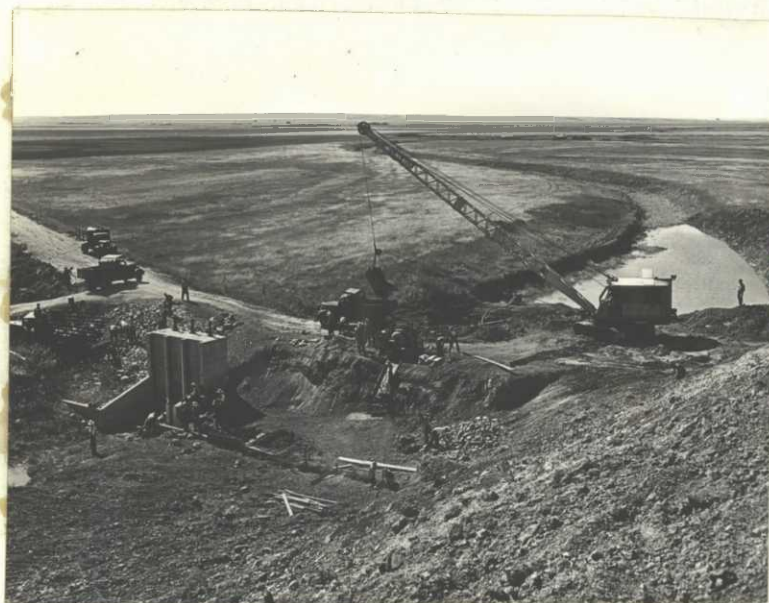
Excavating at #1 Structure preparatory to building overflow spillway.
