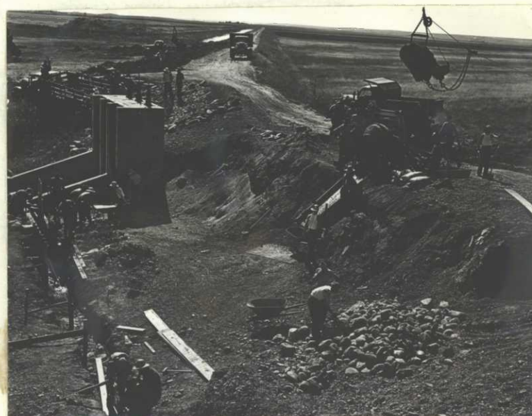
Pouring cutoff wall on #1 overflow structure.
