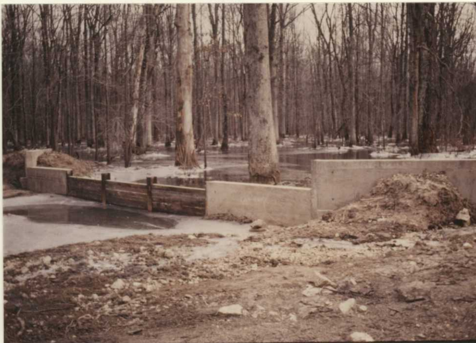
New water control structure in pool 8.
