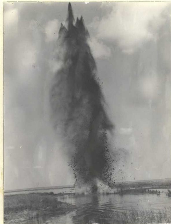
The water and muck was too deep to allow use of the caterpillar so a charge of eight sticks of 40% powder was spread over the spot. The powder lifted the muck out of the water and the wind deposited it high on shore.
