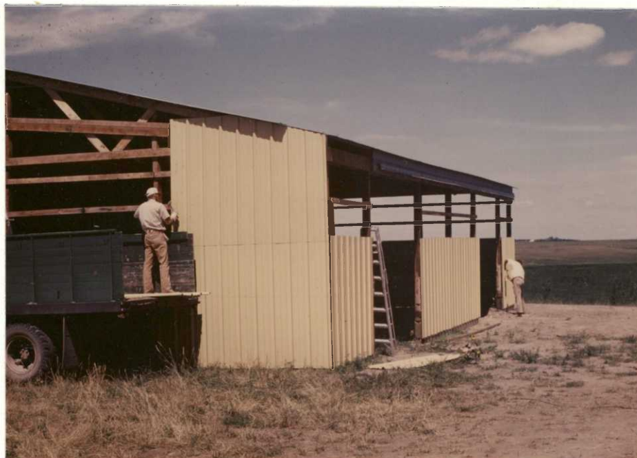
Asst. Manager Fran Maiss (standing on truck bed) and summer employee Gary Brovold putting new siding on 40 ft. x 60 ft. pole building used for equipment storage. #4-80, August 80', H.T. Stone
