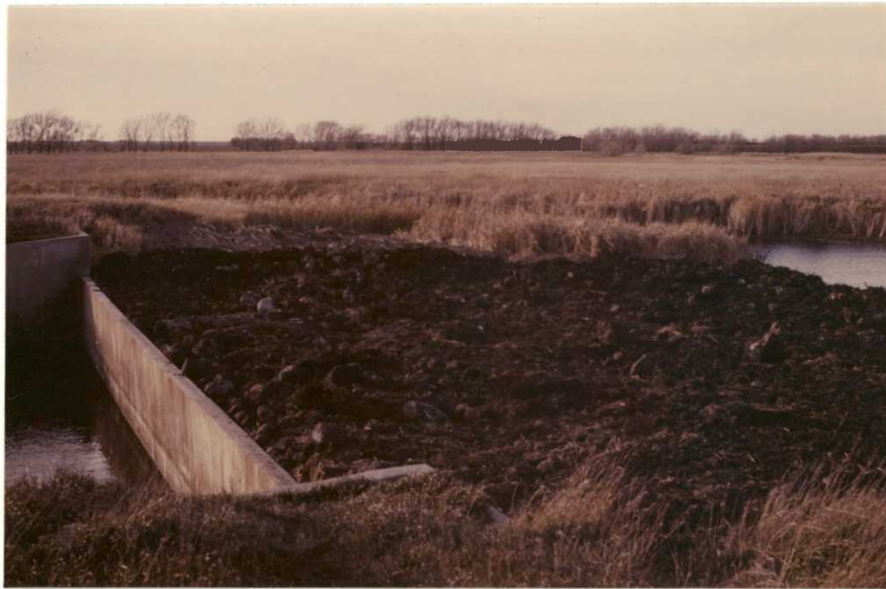
Photo of Maple River Dam spillway after repairs had been completed. Clay fill was packed in behind the concrete wall and then rip-rapped. #10-80, Nov. 5, 1980, H.T. Stone
