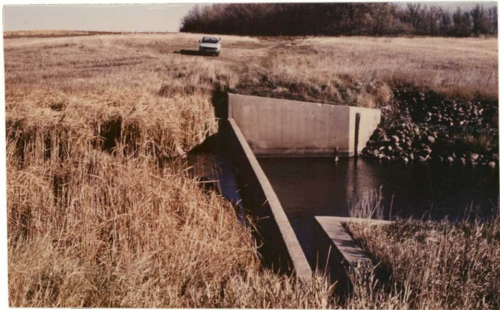
Photo showing the spillway for Maple River Dam before repairs. Note exposed concrete wall from which earthen fill had been washed away. #9-80, Oct. 30, 1980, H.T. Stone
