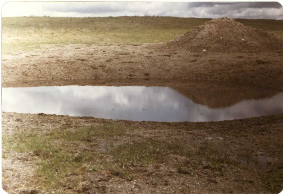
#16 - Spring development on the Baltzer (70) L. A small pond was excavated on gravel soil right over the spring site. 81-16 JWJ
