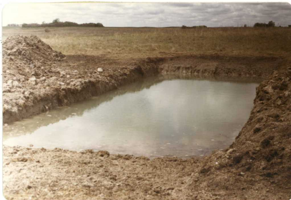
#17 - A small traditional style dugout which collects groundwater on the Kempf (25) McI WPA. 81-17 JWJ
