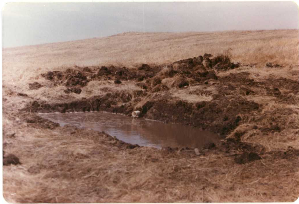
#15 - Spring development on the Werth (166) McI WPA. The spring was excavated to a depth of 6-8 feet, filled with rock and piped about 30 feet down hill to an excavated holding basin. 81-15 FGM
