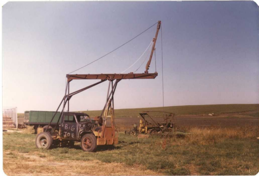
#18 - A boom was constructed and adapted to fit a local wrecking truck (above) so that the pole barn rafters could be lifted by winch cable and set into place (below). 81-19 FGM
