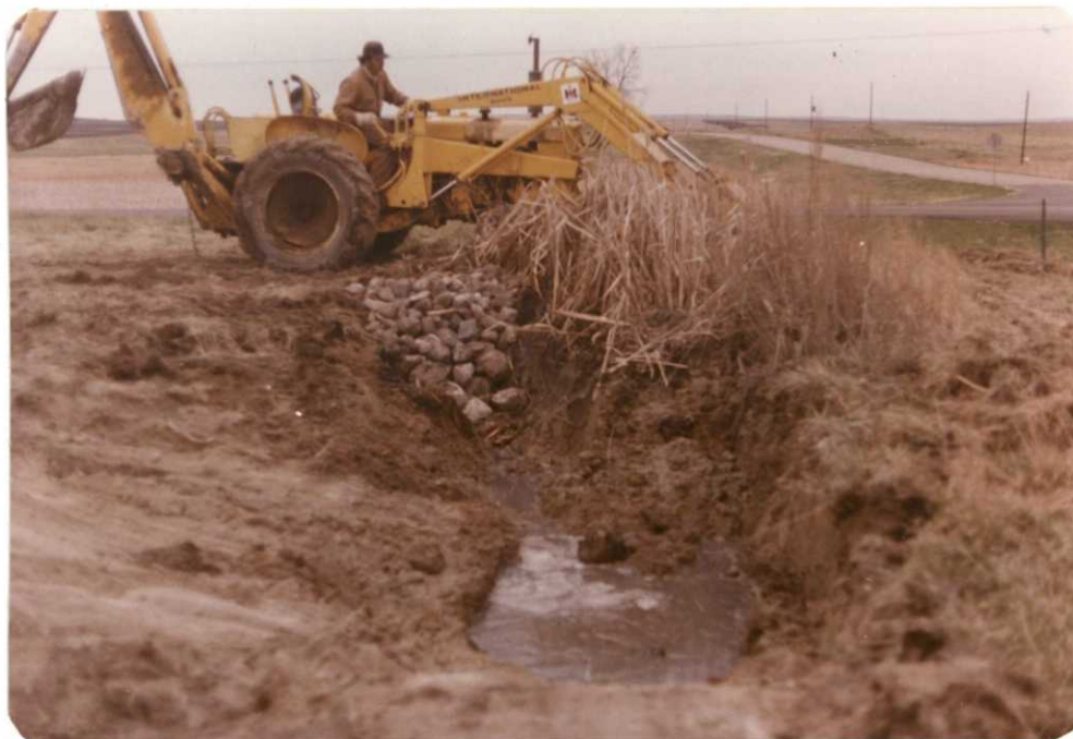
#14 - Spring development on the Schumacher(150) McI WPA. The spring was excavated to a depth of 6-8 feet and filled with rock to prevent plugging. A small adjacent catch basin stores seepage water. 81-14 FGM
