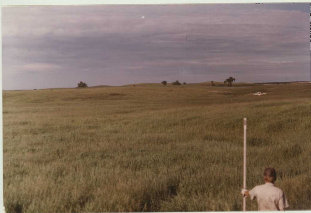
#5 - Level lines were run at the Mund (134) WPA to be certain that the check dam would not flood water through a culvert and onto private land. June 82. LDW
