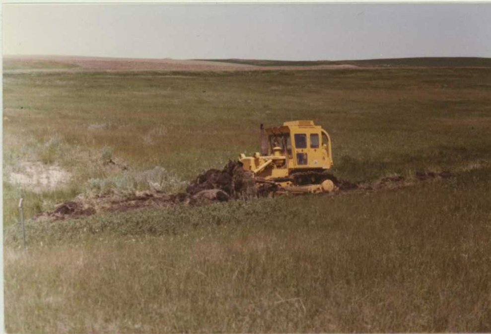
#6 - Dam was constructed at previous ditch cut (left-center) with the loan of a dozer and operator from Sand Lake NWR. July 82. LDW
