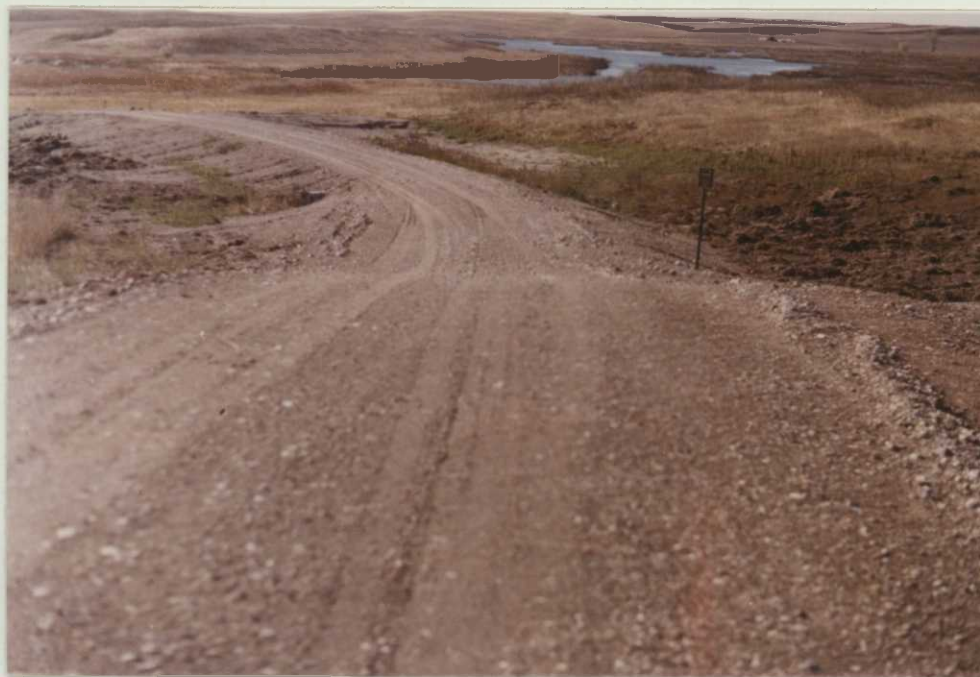
#23 - Gravel was tail gate spread by Kulm personnel from an existing gravel pit on the WPA and road was graded by Logan County. Nov. 82. LDW
