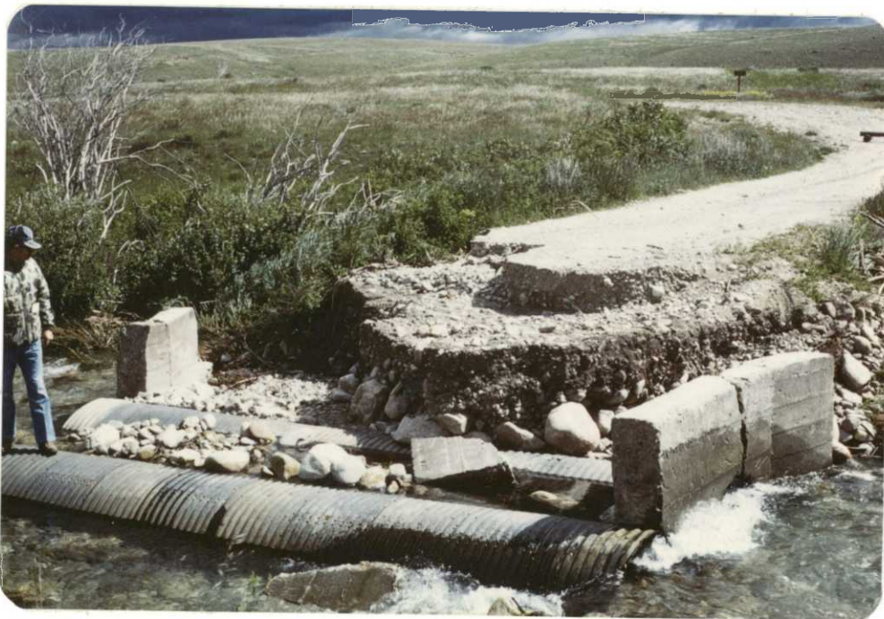
When Flat Creek receded after a week, our west crossing was severely damaged and one culvert washed several hundred yards downstream. (35 mm slide file, 6-16-81, JEW).
