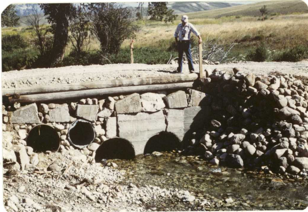
Robbins inspecting repairs. The addition of another culvert, raising the roadbed and providing a deeper emergency spillway to left should save it in the next flood. (35 mm slide file, 7-10-81, JEW).
