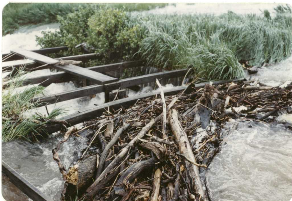
Irrigation structures near Flat Creek clogged with run-off debris (west of McBride shed). (35 mm slide file, 6-10-81, JEW).
