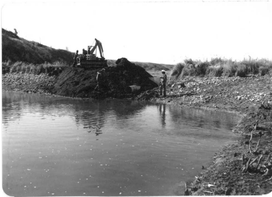
Refuge crew installing 24 inch CMP with anti-seep plate in Pierre's Pond dike washout. (Roll 197-9, 10-16-81, JEW).
