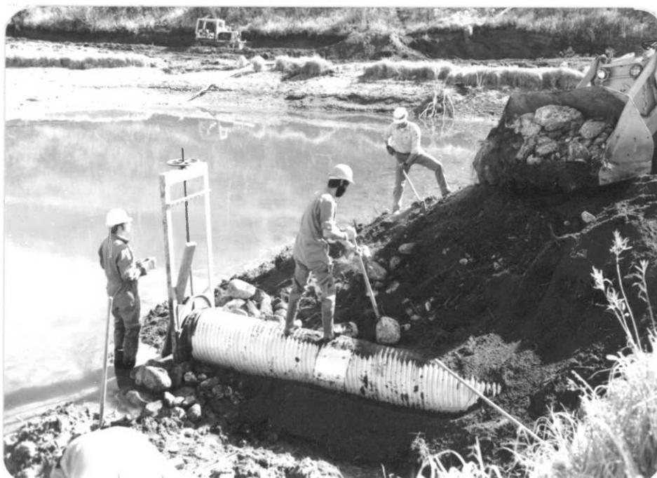
Control gate on 24 inch CMP will allow some control over water levels and occasional drawdowns. Borrow for dike plug taken from base of hill in background (left to right: Griffin, Ryan, Pape). Roll 197-11a, 10-16-81, JEW).
