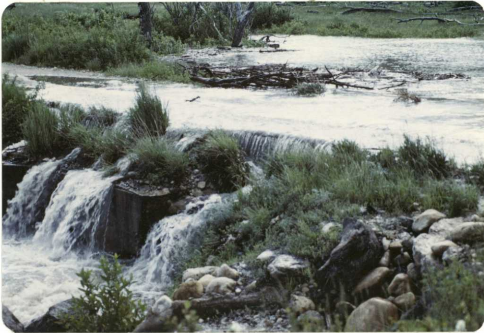
The west crossing on Flat Creek. Culverts couldn't handle and creek over-topped roadway. (35 mm slide file, 6-19-81, JEW).
