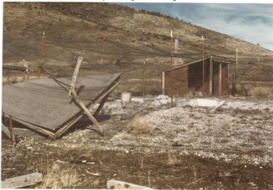
The old raptor pen was mostly destroyed during the August fire.
