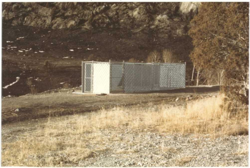
Nearly completed, the new raptor pen was filled with slats to reduce visibility and consequently disturbance to birds. Slats also slow wind velocity and shelter the birds during rain and snow storms. FWC 10/79
