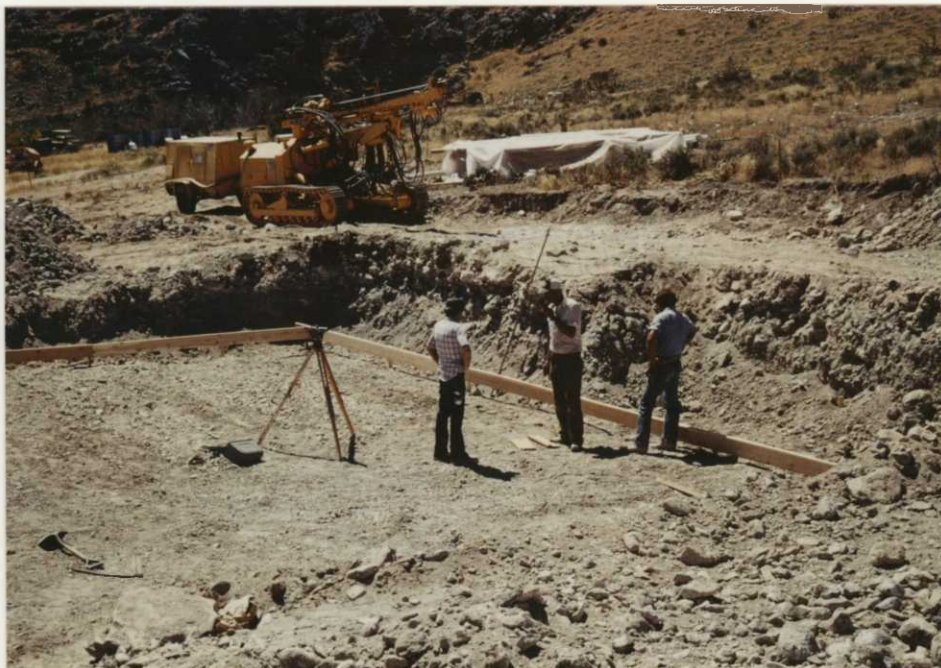
A hill site immediately north of existing headquarters building was chosen for the two new homes and common garage. Here, with the aid of two weeks blasting, excavation for the basement in Quarters # 100 is complete.
