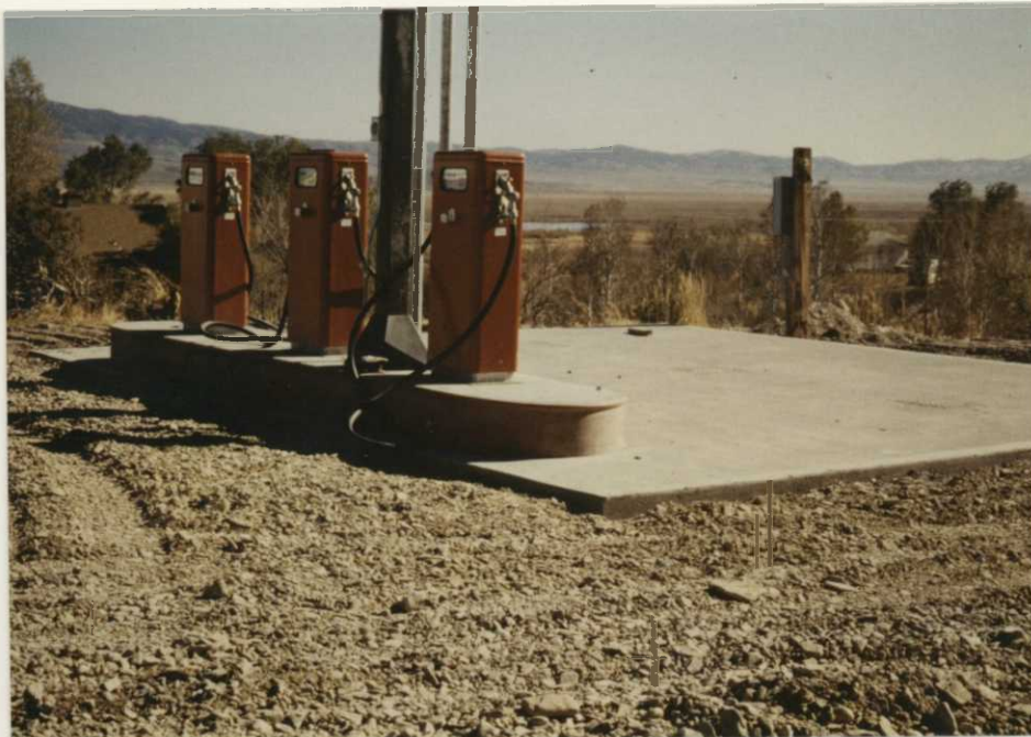
Fuel service island was moved from immediately behind the office to a safer location above the shop. Facility consists of three 1,000 gallon fiberglass tanks, each with a new Wayne pump. Electrical service, upper right, was designed to eventually accommodate a new oil storage building. FWC 10/80
