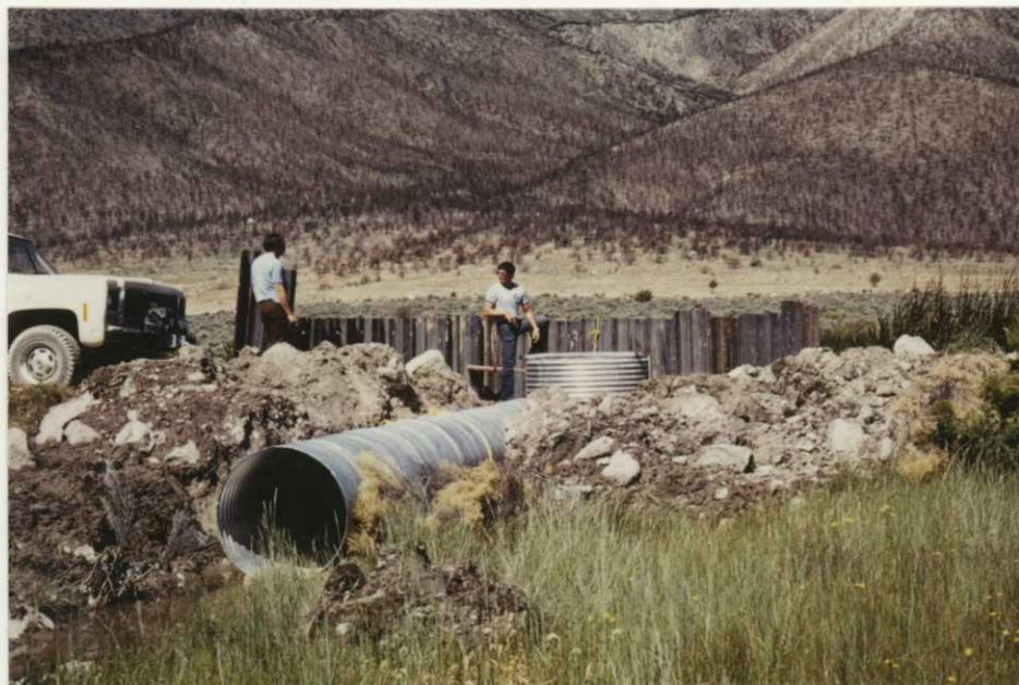
Bouffard, left, and Cameron discuss installation level of new control structure from the Collection Ditch directly to the North Sump. DNJ 8/80
