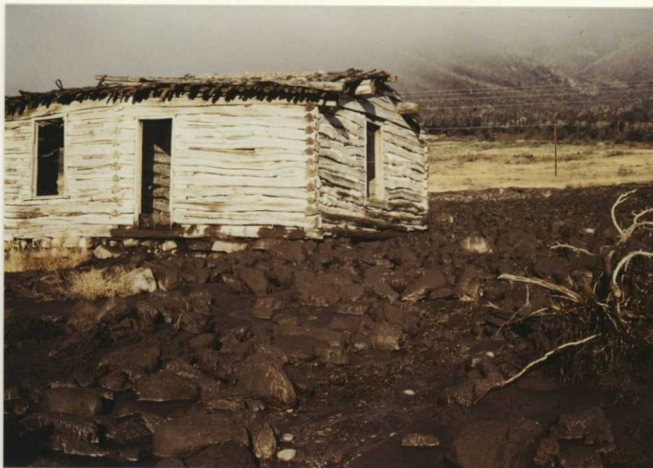
On 7 September, 1980, heavy rains on the watershed of the 1979 Shantytown burn, see canyon in upper right, washed large boulders into the foundation of Bressman cabin. Rocks caused structural damage to the west (back) wall of the old settlers cabin. DNJ 9/8/80
