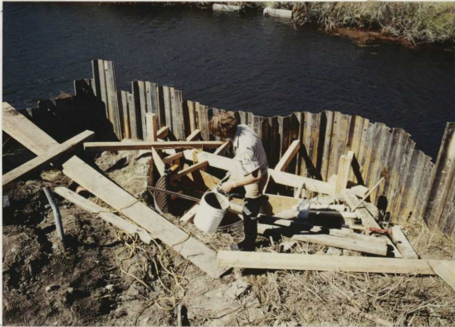
Bowser begins cementing process to insert and seal a CMP riser into an old crumbling concrete headwall.
