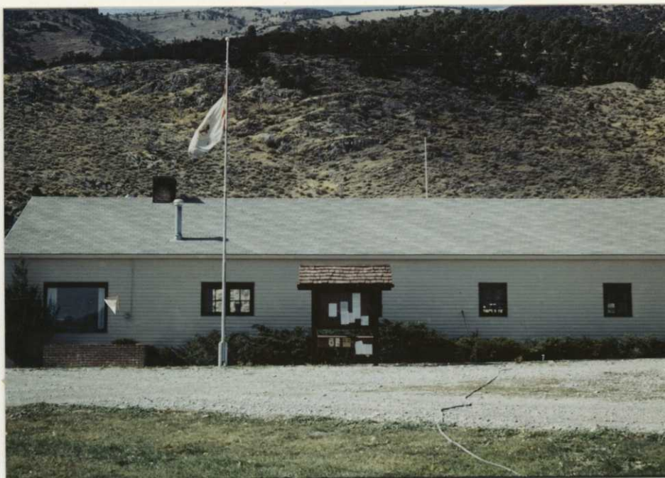
In this 1978 photo, the 1941 office was still doubling as a shop. The entrance was at the left end of the building and office space was 14'x24' and included a restroom, office, reception and clerical area. Four garage bays made up the rest of the building. MDS 9/78
