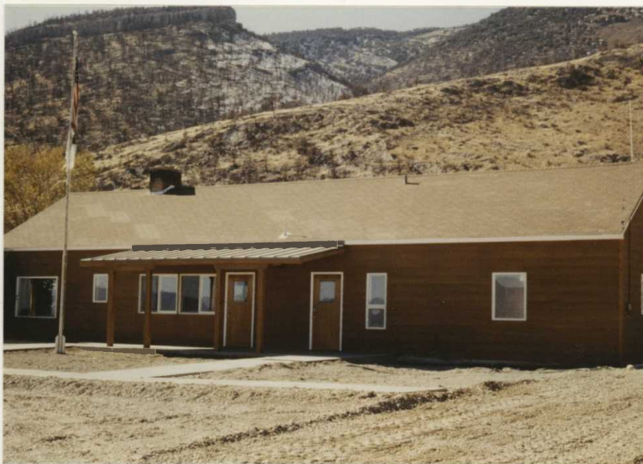
After 1980 construction, the entrance was in front with level, gravelled parking area, and a lawn area. Interior consists of seven rooms and a single garage stall. The new heating system and insulation seems to use no more energy to heat four times the space. FWC 10/80
