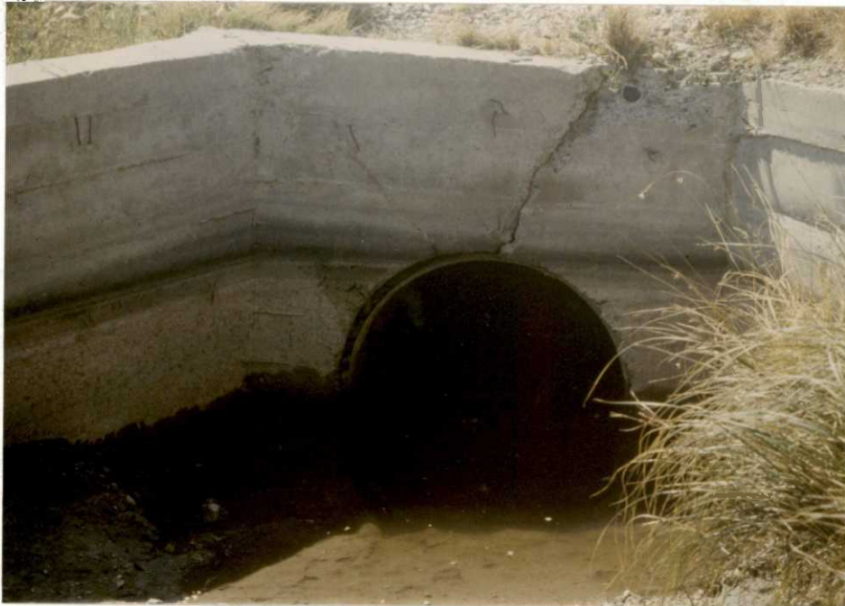
Repairs were required because of cracked headwalls and stop-log channels, or because of poor design with stop-log channels too close to headwalls allowing pondweed to clog the flow. FWC 6/79
