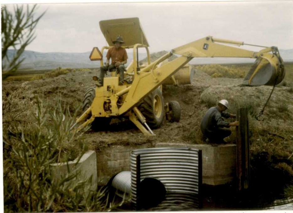
Henry and John Krenka placed coffer dams around the structures so the area could be pumped dry to pour concrete around CMP insert. FWC 7/81
