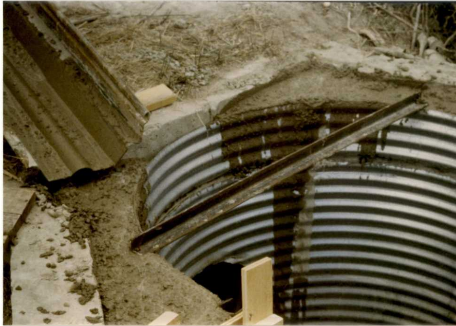
Sakrete was mixed since no redimix is available. A new 30" riser with 60" stoplogs was inserted against the old headwall and into the old 36" culvert. The reduced volume will not be critical. FWC 7/81
