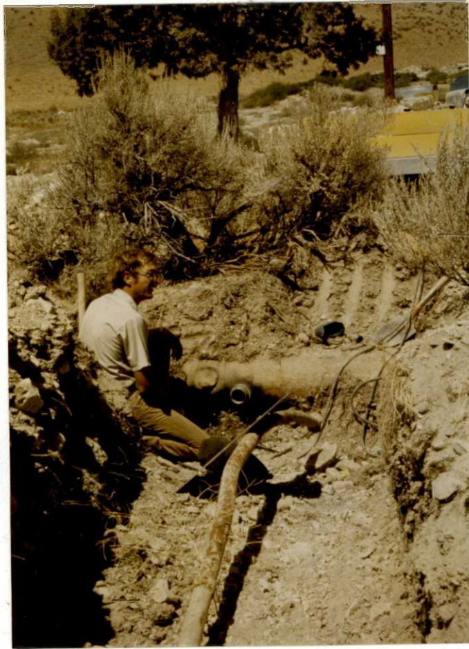
Maintenance mechanic Bowser modifies plumbing near the weather station to more efficiently irrigate the headquarters area. FWC 6/82
