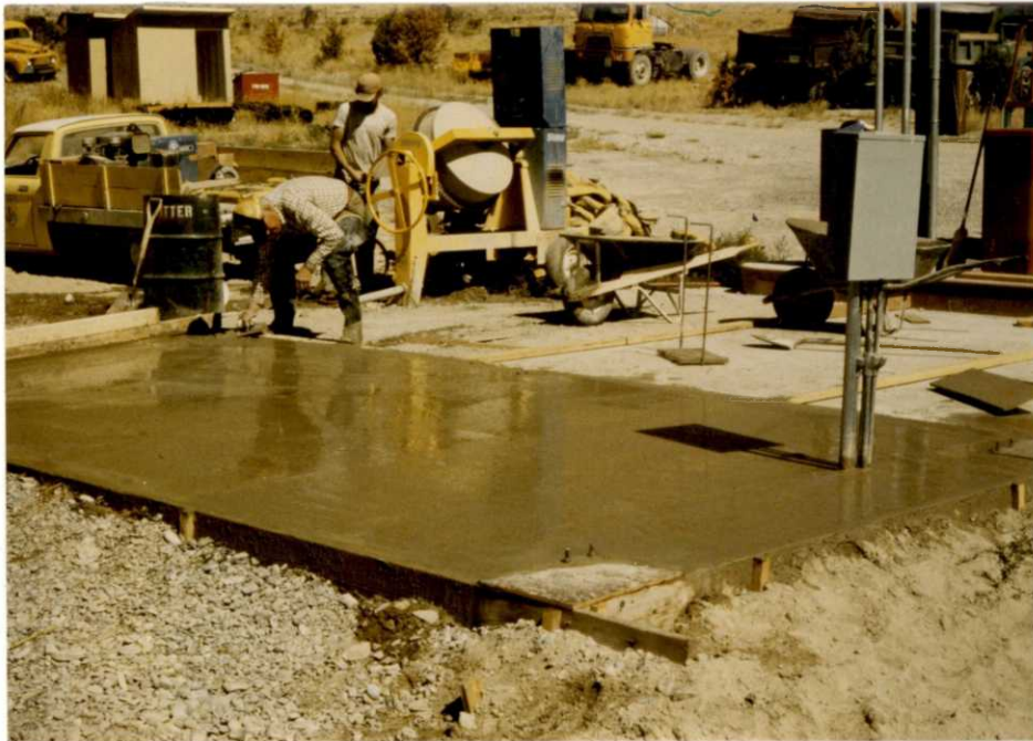
Marsh and Butler put finish on slab for our new oil storage building. Since no redimix companies care to deliver into Ruby Valley, it takes a lot of Sakrete. 8/81 FWC
