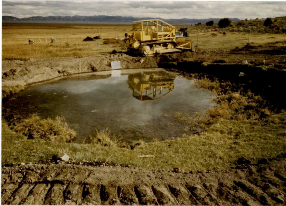
Here a watergap is being completed in the County Line area. The springhead was fenced off for protection and a float-operated tank supplies water to cattle grazing on adjacent Forest Service land. FWC 9/81
