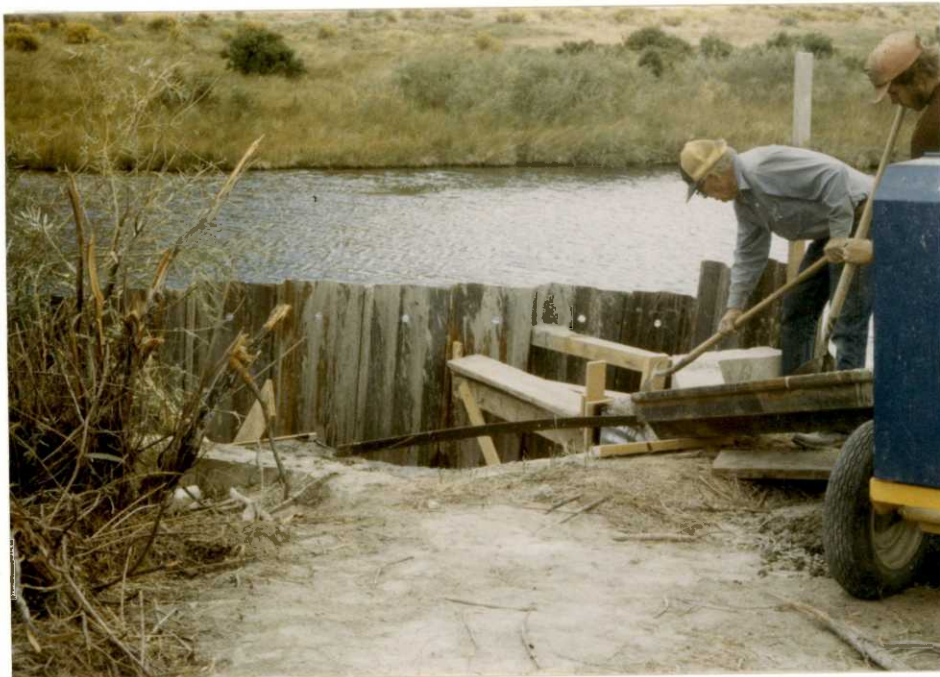
Howell Marsh and YACC David Butler made forms and poured concrete to join the new CMP riser to the old headwall. FWC 7/81
