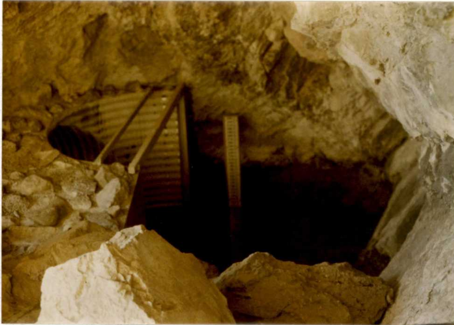
The finished structure was faced with native stone for aesthetics and the old plywood and timber flow gate was removed. FWC 7/81
