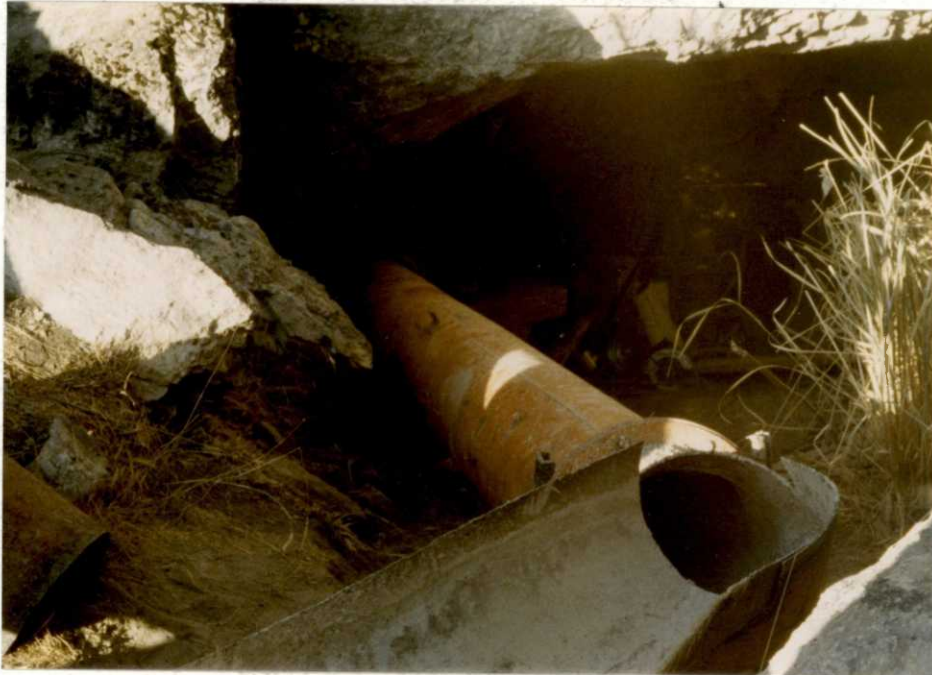
Placing the structure inside the cave at the head of Cave Creek required this elaborate concrete chute. Concrete was poured in water flows of 4 cfs. FWC 7/81
