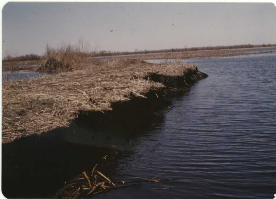
Dike erosion north of Pintail Point where rip-rap project failed last year. 11/82 BH
