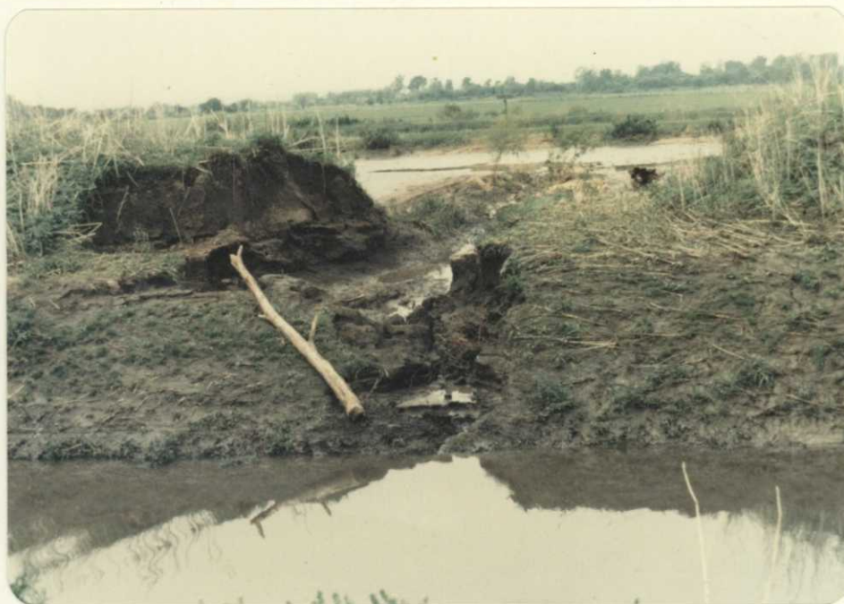
June washout in the west levee of Squaw Creek one-fourth mile north of the Napier Bridge. 6/82 BH
