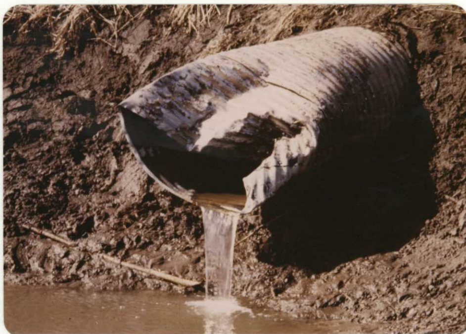
Inflow tube (3') for Mallard Marsh crushed by ice breakup on Squaw Creek in February. 2/82 BH
