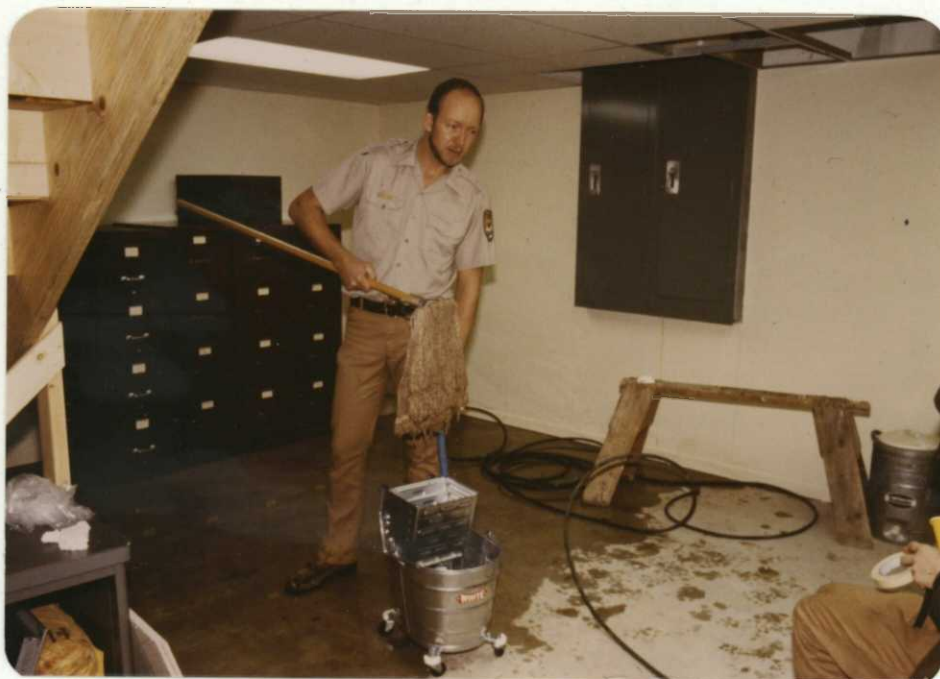
Grannemann mans the mop after a shower brought water into the basement. It came in above the panel boxes and ran down inside and outside the insulated wall. 7/82 BH
