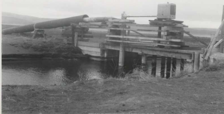
8. Temporary pump installation to irrigate land in Secs. 18 & 19, Twp. 48 N., R. 2 E., just south of State Line Highway. (Ramelli)
