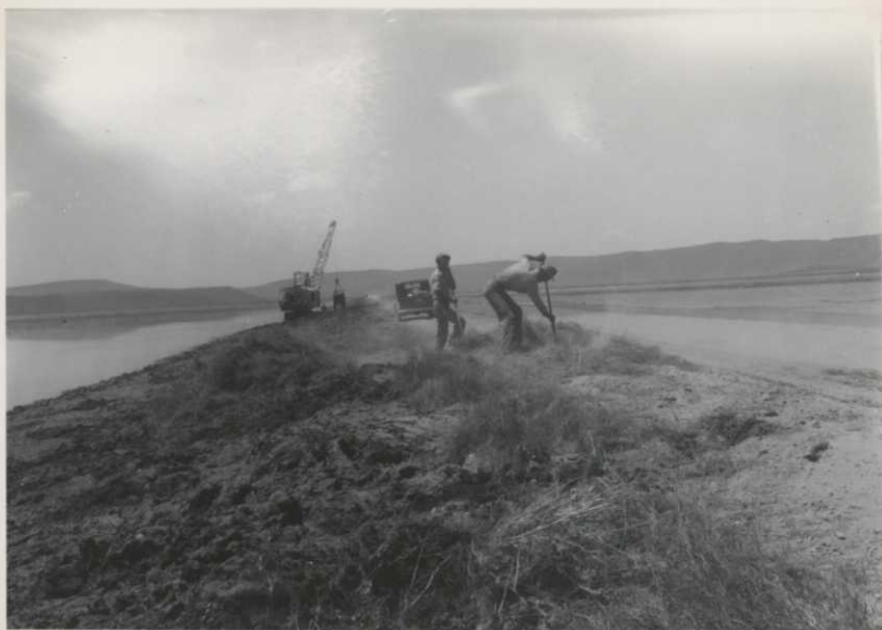
5. Cleaning weeds off dike preparatory to dragging. (Ramelli)
