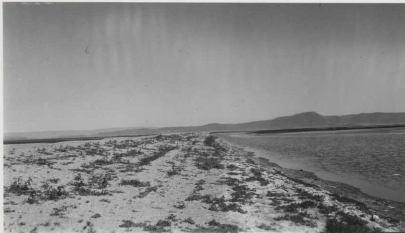
7. Dike slope after dragging and seeding. Fair to good stand of grass (Crested wheat, Italian Rye) and Sweet clover (white & yellow) on upper slope. Scirpus paludosus and water millet seeded along toe. (Sargeant)
