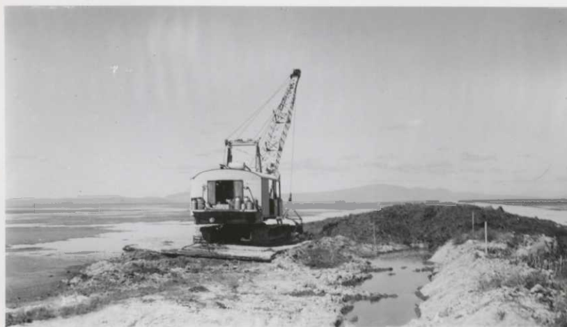
4. Dragline at work on lower end of Unit 4 dike - borrowing from Unit 7 side. Limited amount of old dike left in place to provide solid core. (Sargeant)
