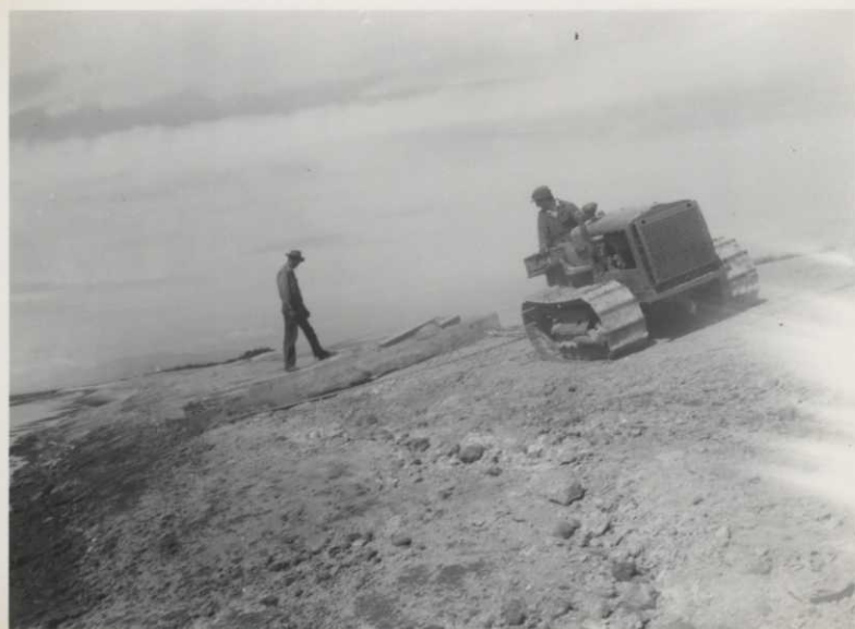
6. Dragging dike slope preparatory to seeding. ("22" Cat. and refuge constructed drag.) (Ramelli)
