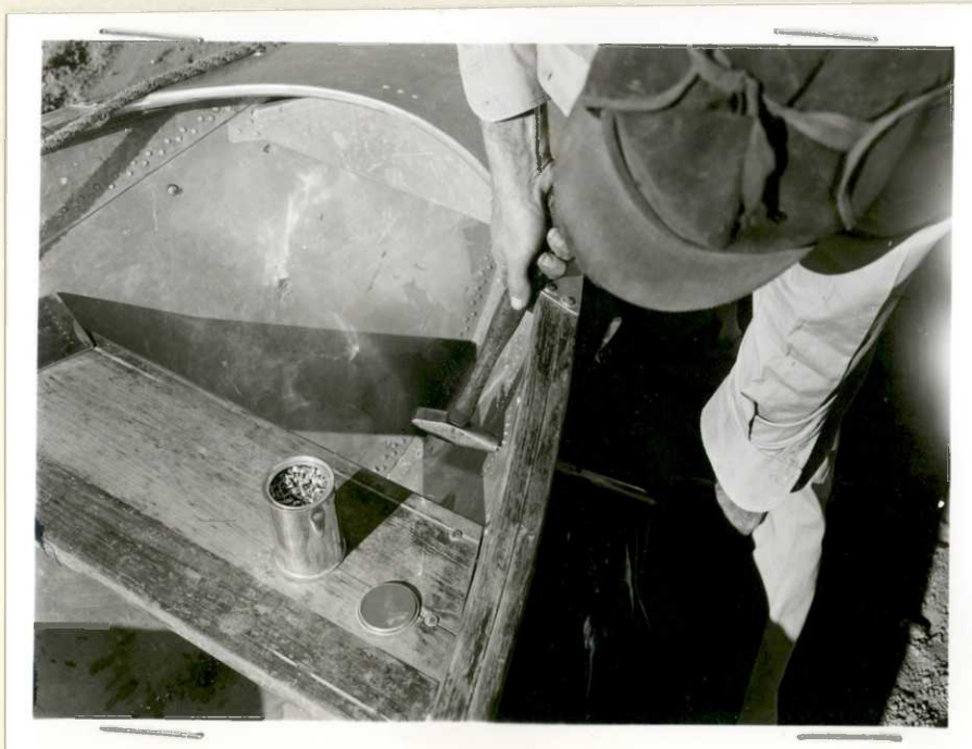
Riveting the letters FWS with hammer and bucking bar.
