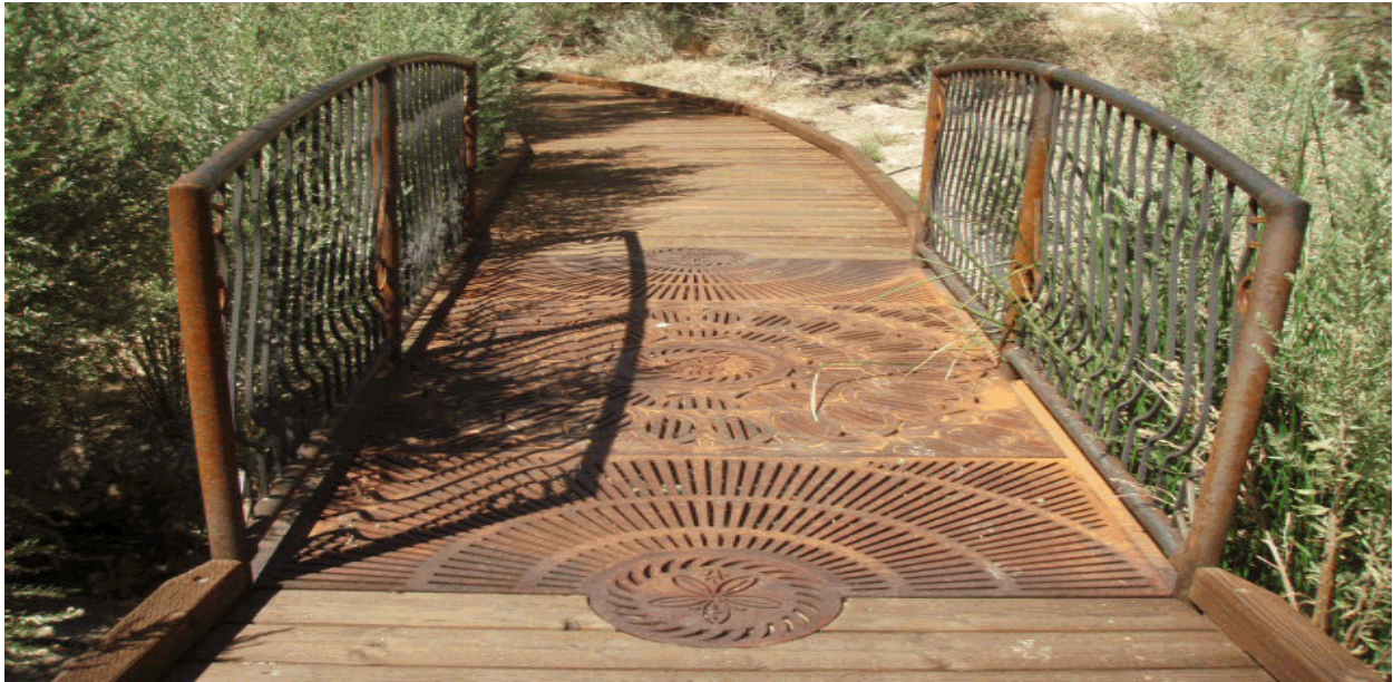
Photo # ASME_C2_1100 - MP 0.11 - Bridge -sf
