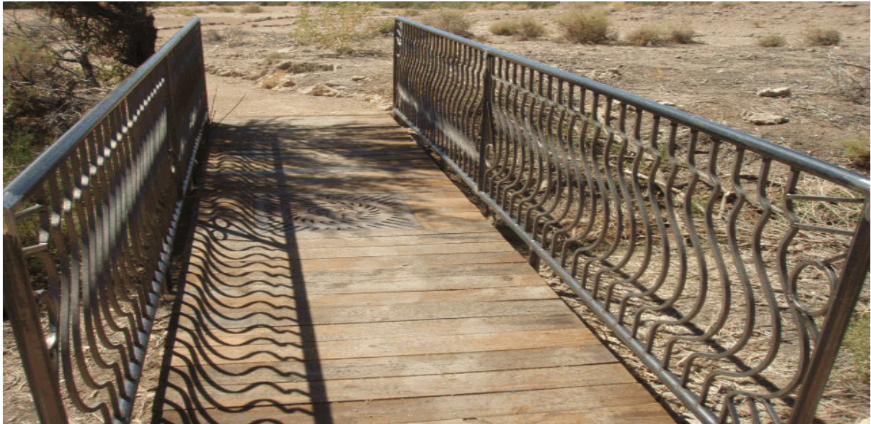
Photo # ASME_C2_1097 - MP 0.19 - Bridge -sf
