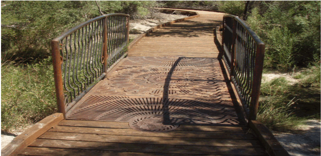
Photo # ASME_C2_1093 - MP 0.09 - Bridge -sf
