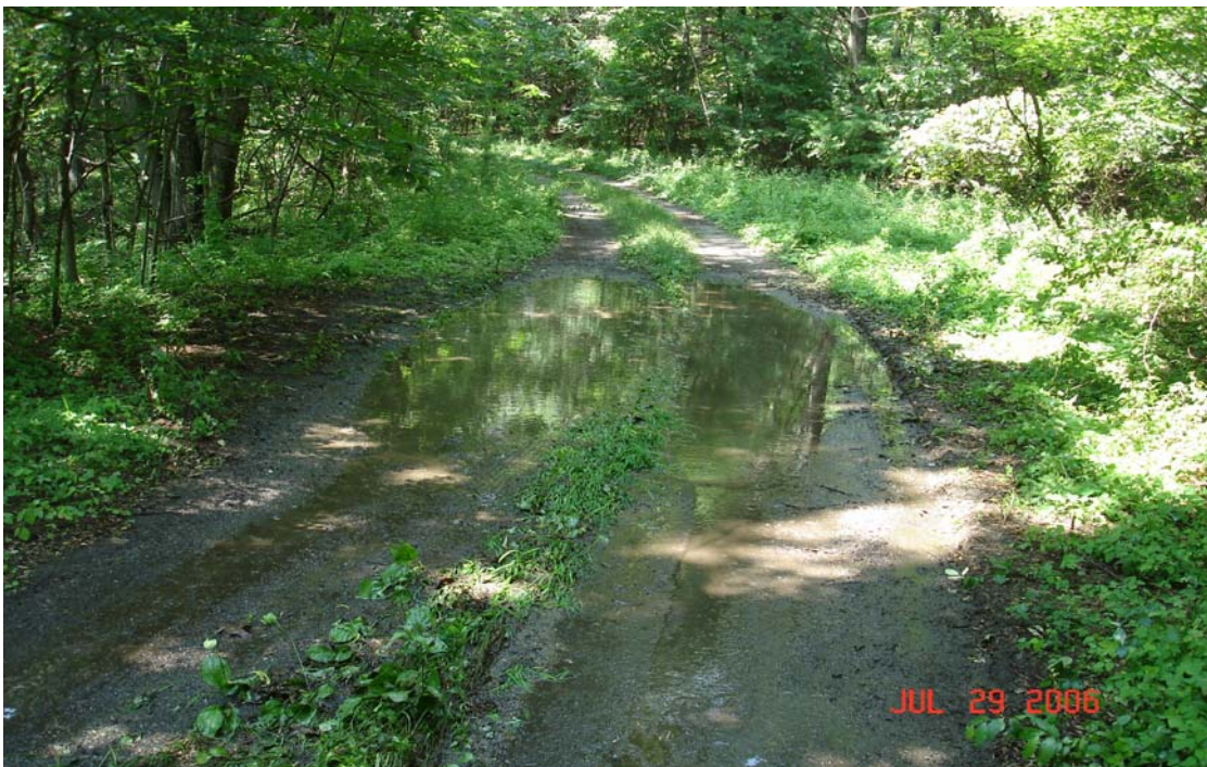
Photo # 12 - MP 1.77 - Drainage Deficiency
