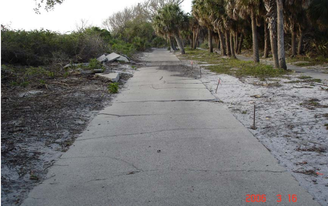
Photo # 49 - MP 0.0 - Trailhead, Trail Structure Deficiency (Broken Concrete)
