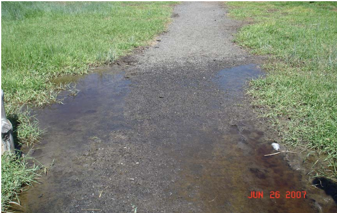
Photo # 118 - MP 0.11 - Drainage Deficiency
