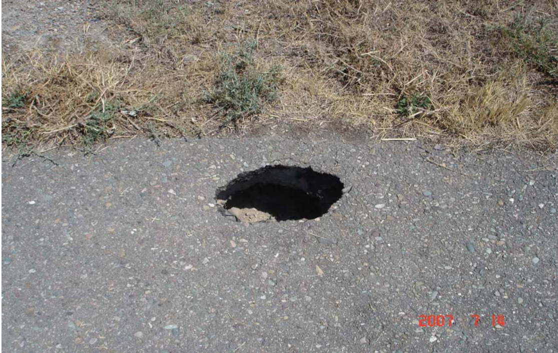
Photo # 6 - MP 0.16 - Erosion Deficiency
