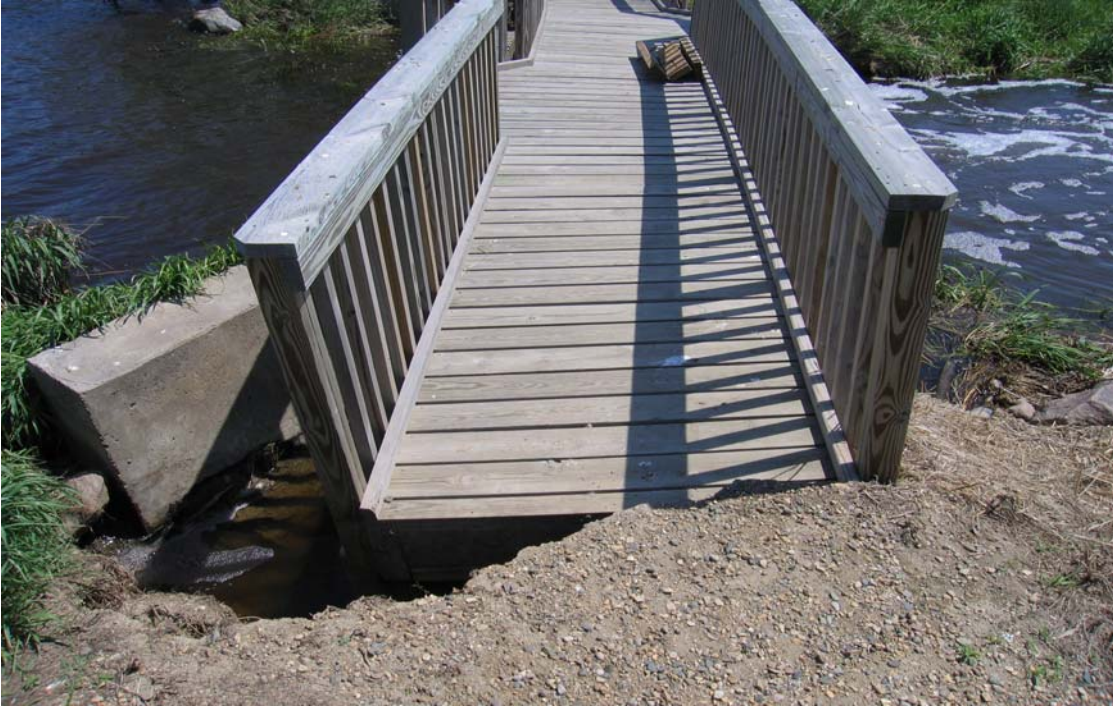
Photo # 1612 - MP 0.88 - Trail Structure Deficiency, Bridge
