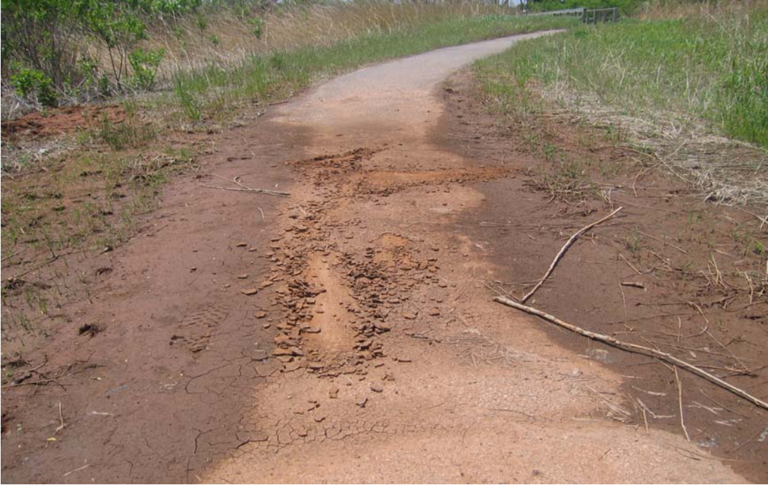
Photo # 0864 - MP 0.09 - Drainage Deficiency
