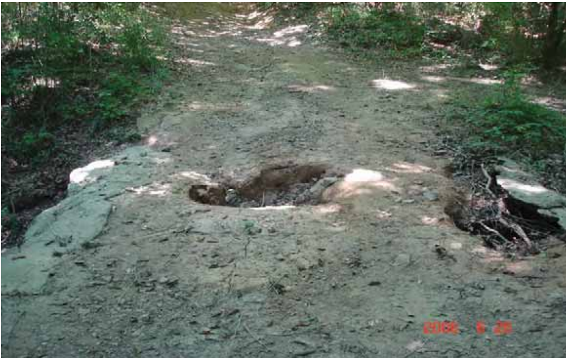
Photo # 5 - MP 1.79 - Drainage Deficiency
