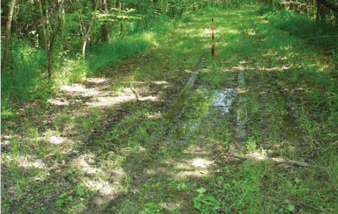
Photo # 83 - MP 0.21 - Drainage Deficiency
