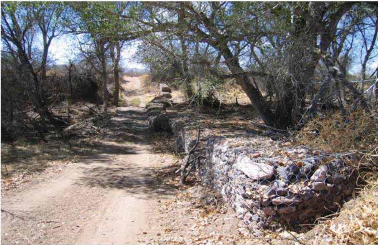
Photo #0081- MP 1.56 - Crib Wall-Rock
