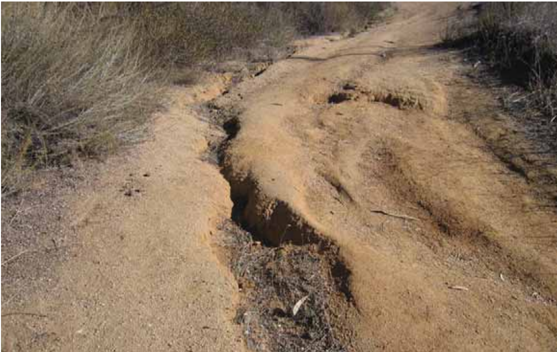
Photo # 2091 - MP 0.07 - Erosion Deficiency
