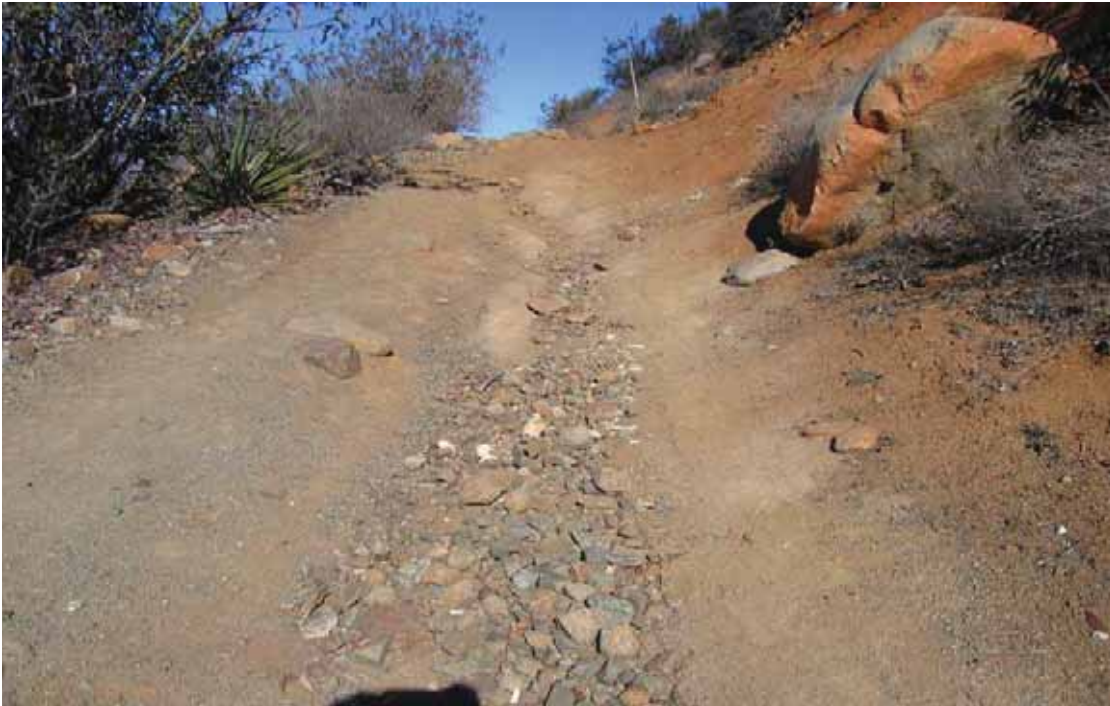
Photo # 2102 - MP 0.79 - Erosion Deficiency
