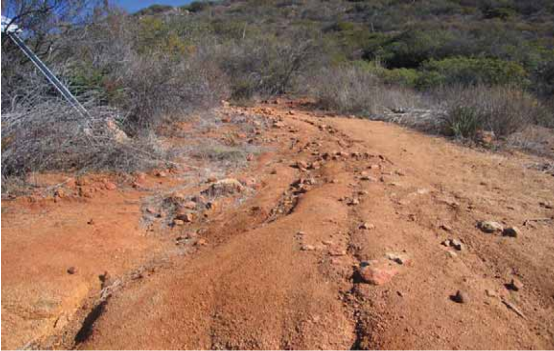
Photo # 2094 - MP 0.34 - Erosion Deficiency, Begin Section 002
