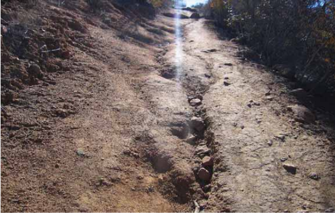
Photo # 2096 - MP 0.48 - Erosion Deficiency
