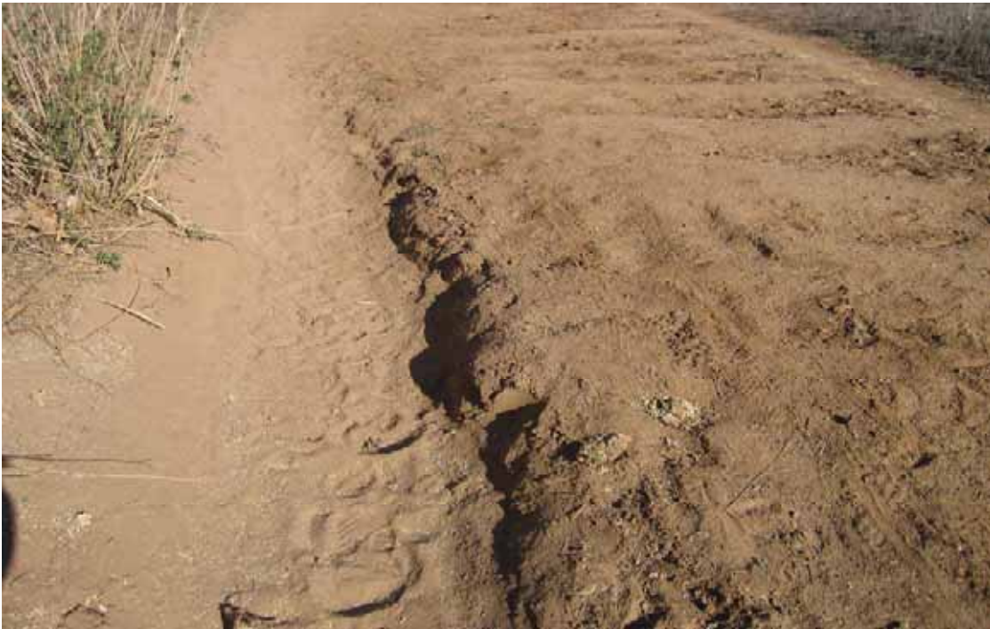
Photo # 2110 - MP 0.97 - Erosion Deficiency
