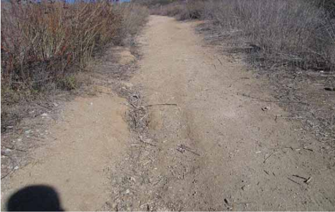
Photo # 2092 - MP 0.17 - Erosion Deficiency
