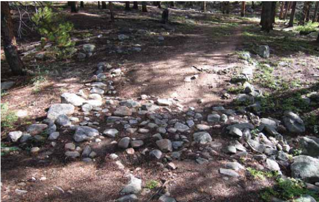
Photo # 2111 - MP 1.33 - Check Dam: Rock
