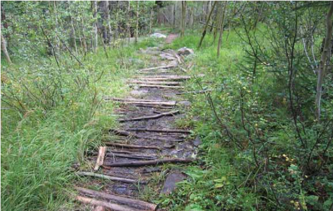
Photo # 2201 - MP 0.95 - Drainage Deficiency
