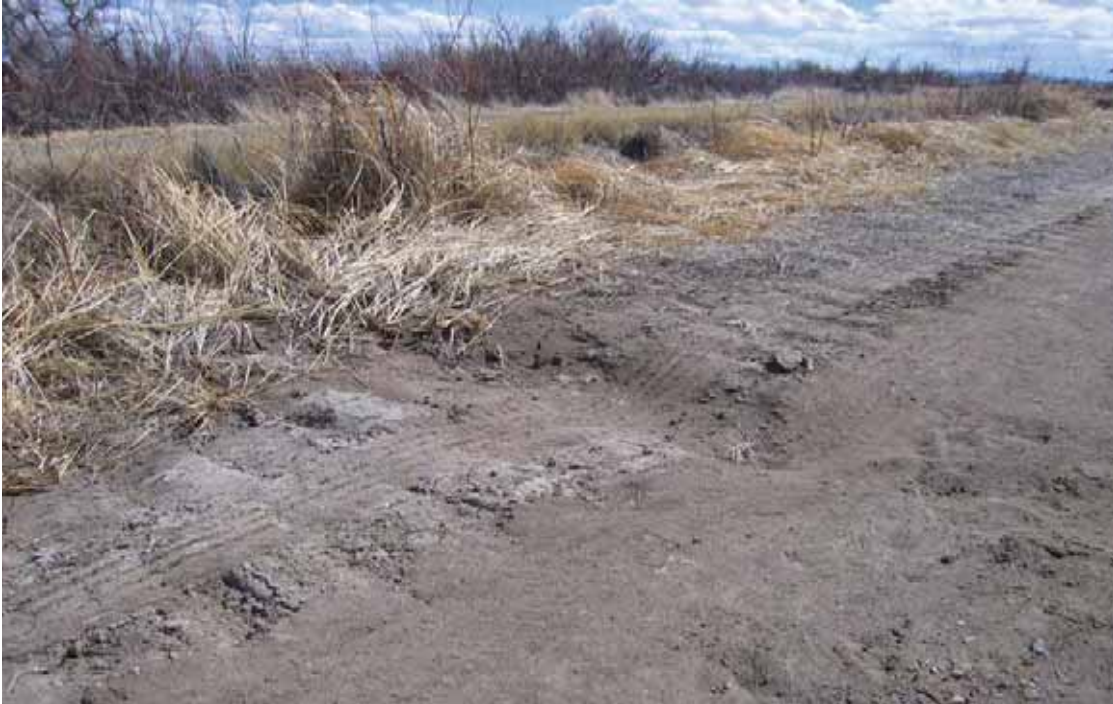
Photo # 2173 - MP 1.8 - Erosion Deficiency
