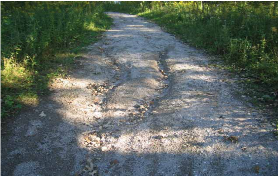
Photo # 0864 - MP 0.09 - Erosion Deficiency
