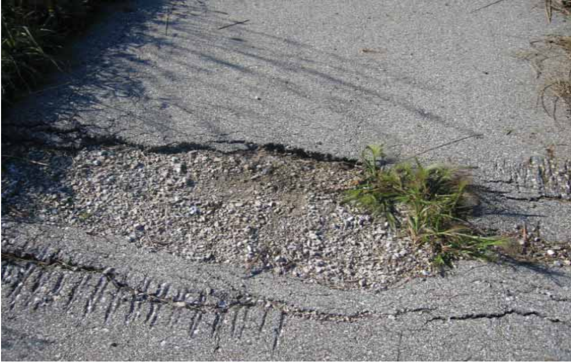
Photo # 0861 - MP 1.24 - Drainage Deficiency
