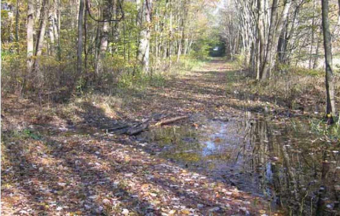
Photo # 1065 - MP 0.15 - Drainage Deficiency
