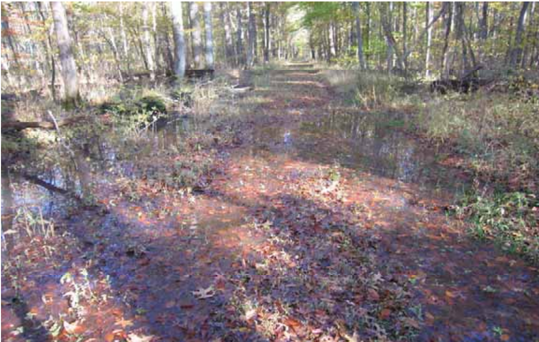
Photo # 1063 - MP 2.17 - Drainage Deficiency
