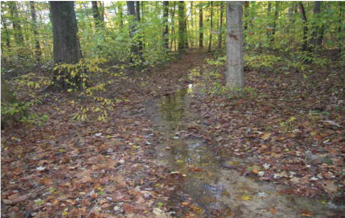
Photo # 1017 - MP 0.13 - Drainage Deficiency
