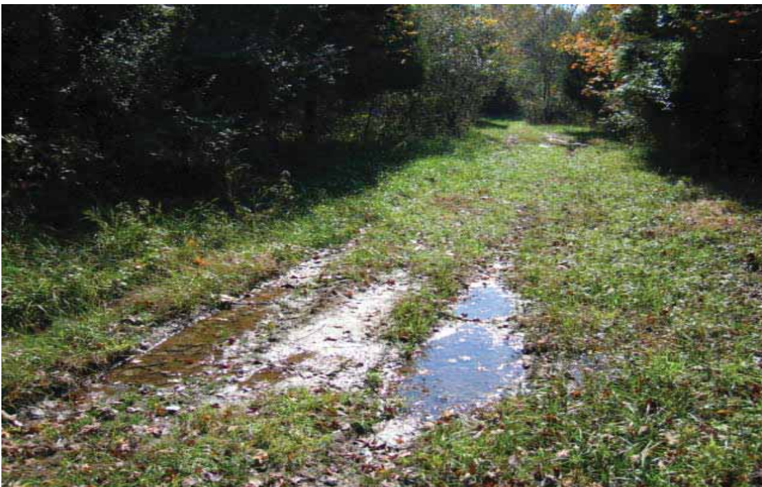
Photo # 1095 - MP 0.08 - Drainage Deficiency
