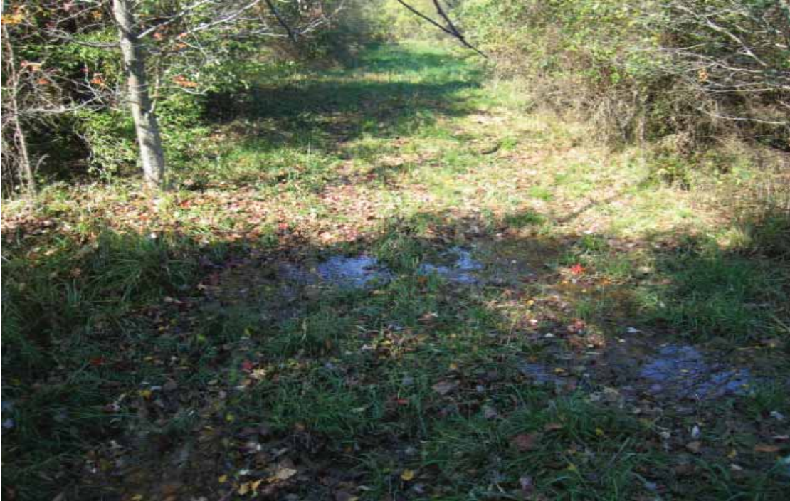
Photo # 1099 - MP 0.18 - Drainage Deficiency
