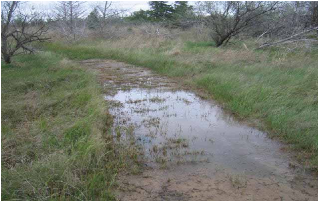
Photo # 1468 - MP 0.2 - Drainage Deficiency
