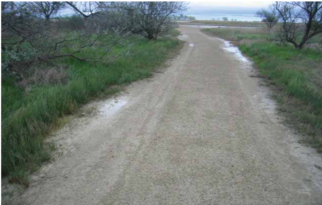
Photo # 1445 - MP 0.04 - Drainage Deficiency
