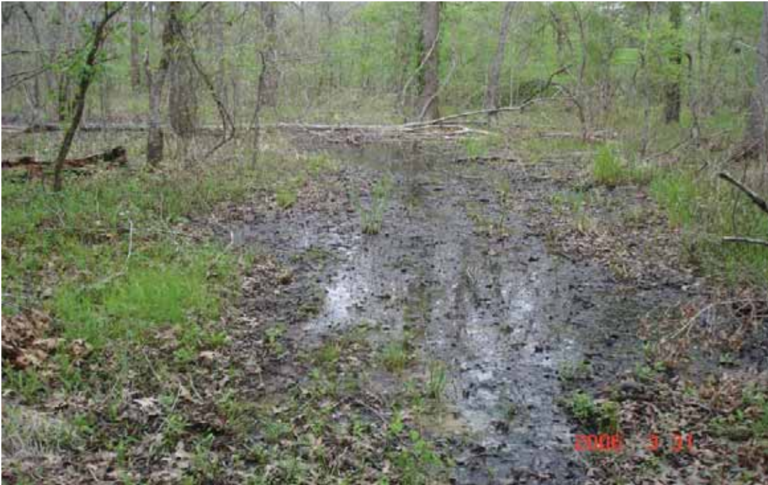
Photo # 44 - MP 1.72 - Drainage Deficiency
