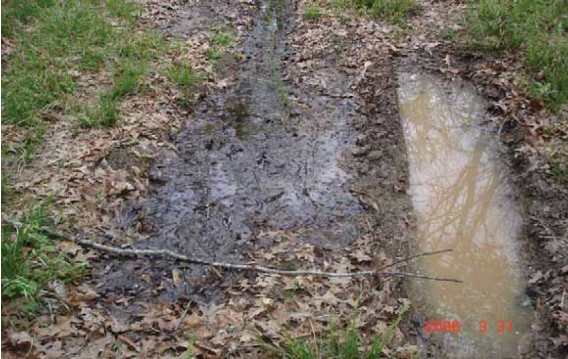
Photo # 27 - MP 0.46 - Drainage Deficiency
