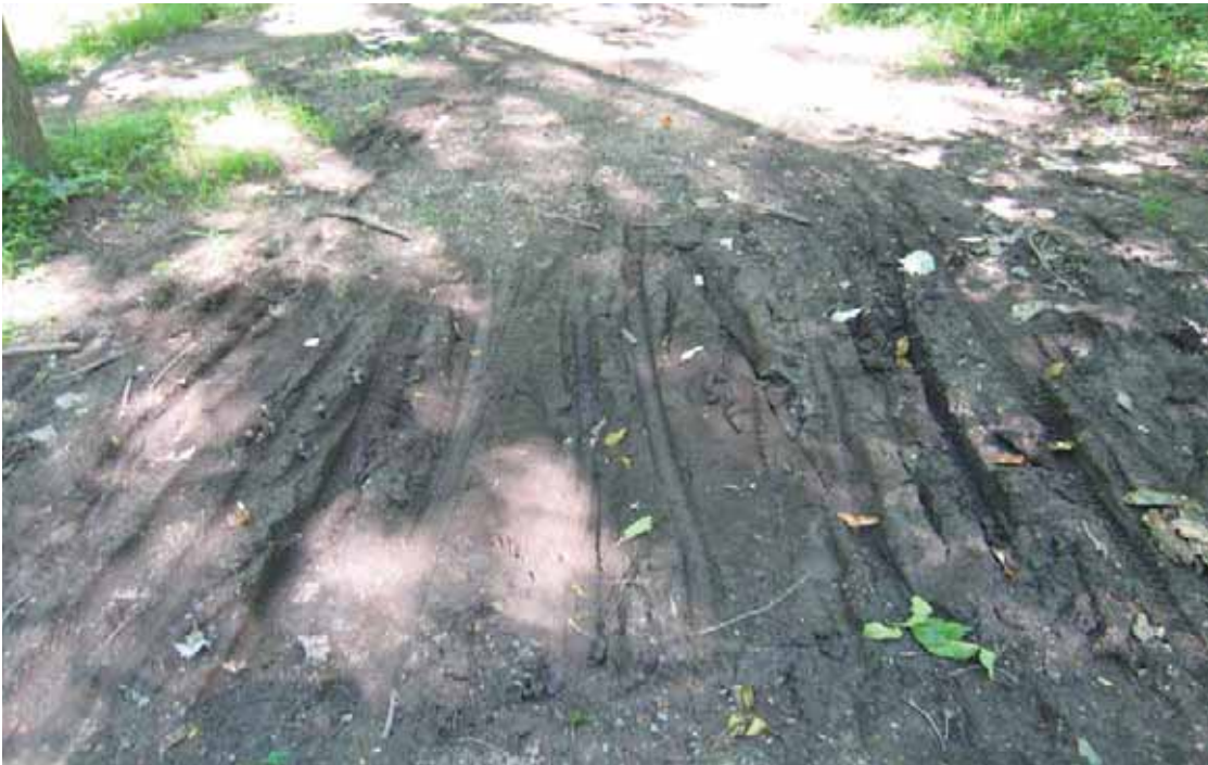
Photo # 1505 - MP 1.48 - Drainage Deficiency
