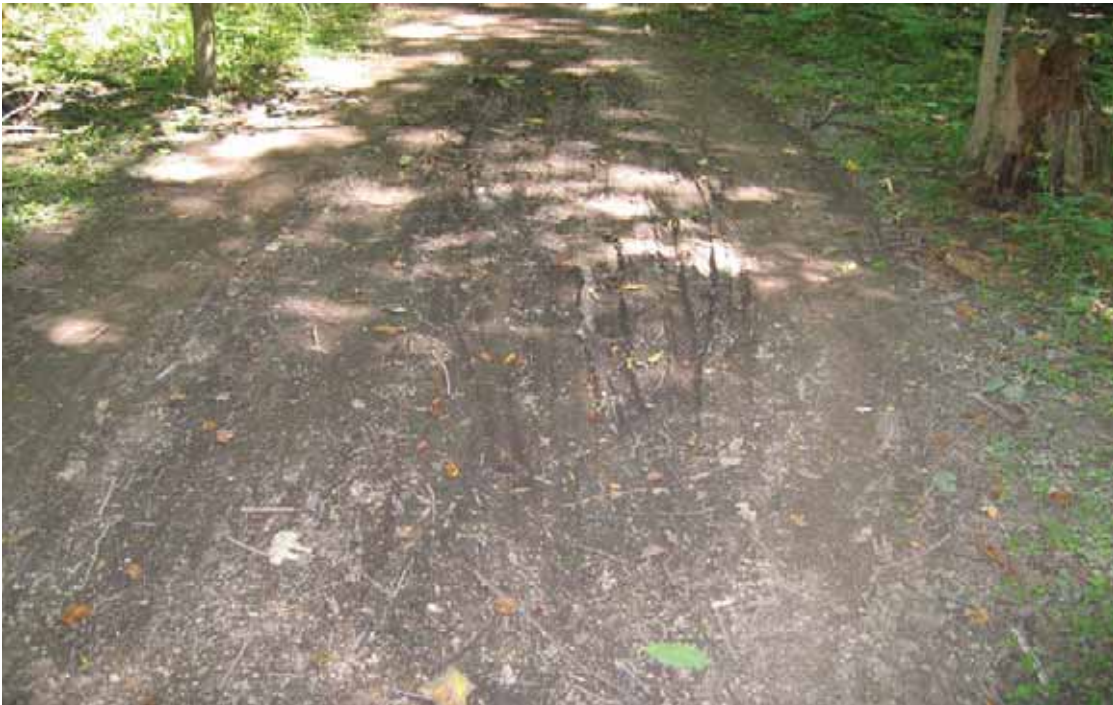
Photo # 1497 - MP 0.87 - Drainage Deficiency
