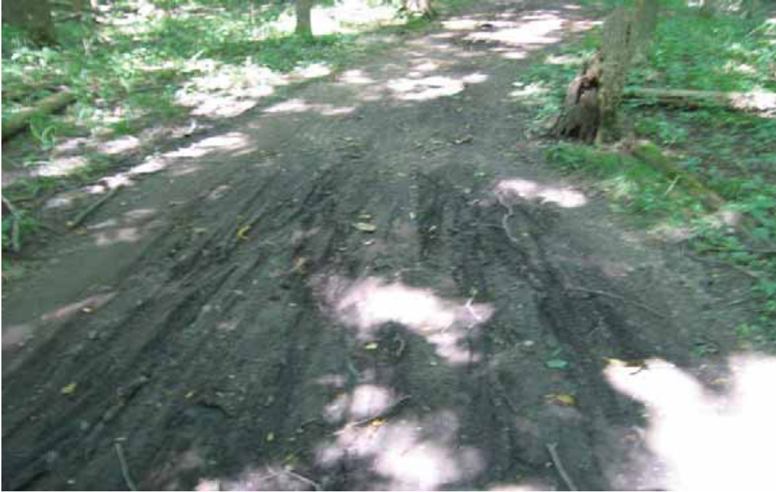
Photo # 1506 - MP 1.64 - Drainage Deficiency
