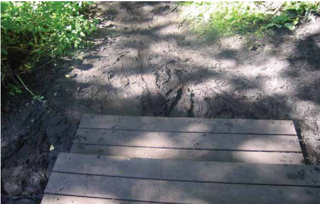
Photo # 0631 - MP 0.15 - Drainage Deficiency
