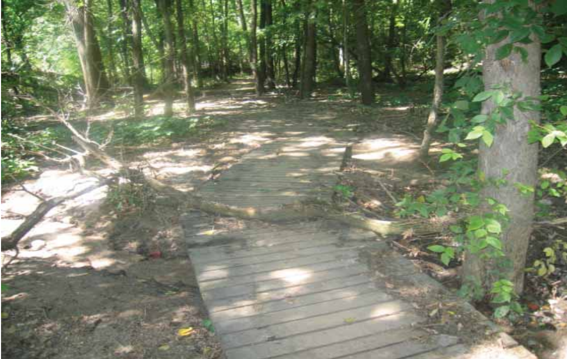
Photo # 0647 - MP 0.58 - Boardwalk, Trail Structure Deficiency
