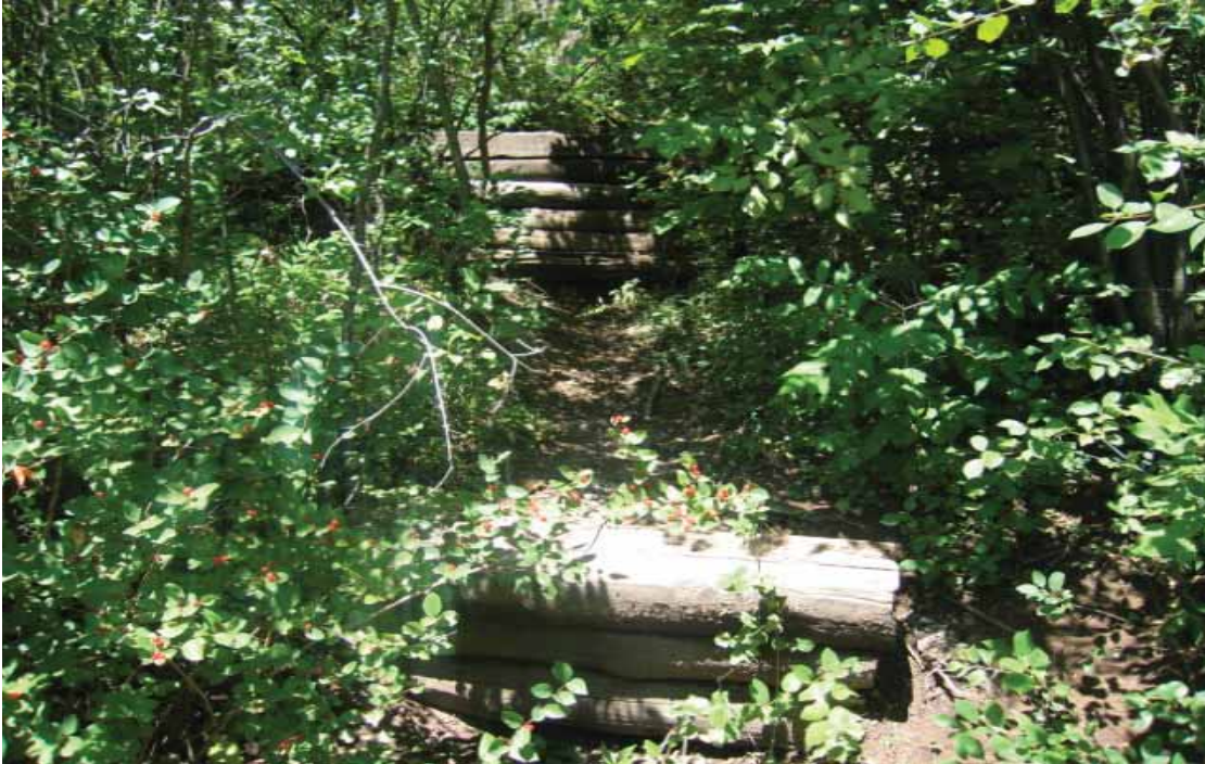
Photo # 0657 - MP 1.48 - Check Dam: Log
