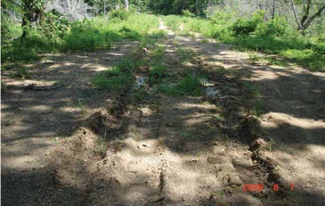
Photo # 19 - MP 0.71 - Drainage Deficiency
