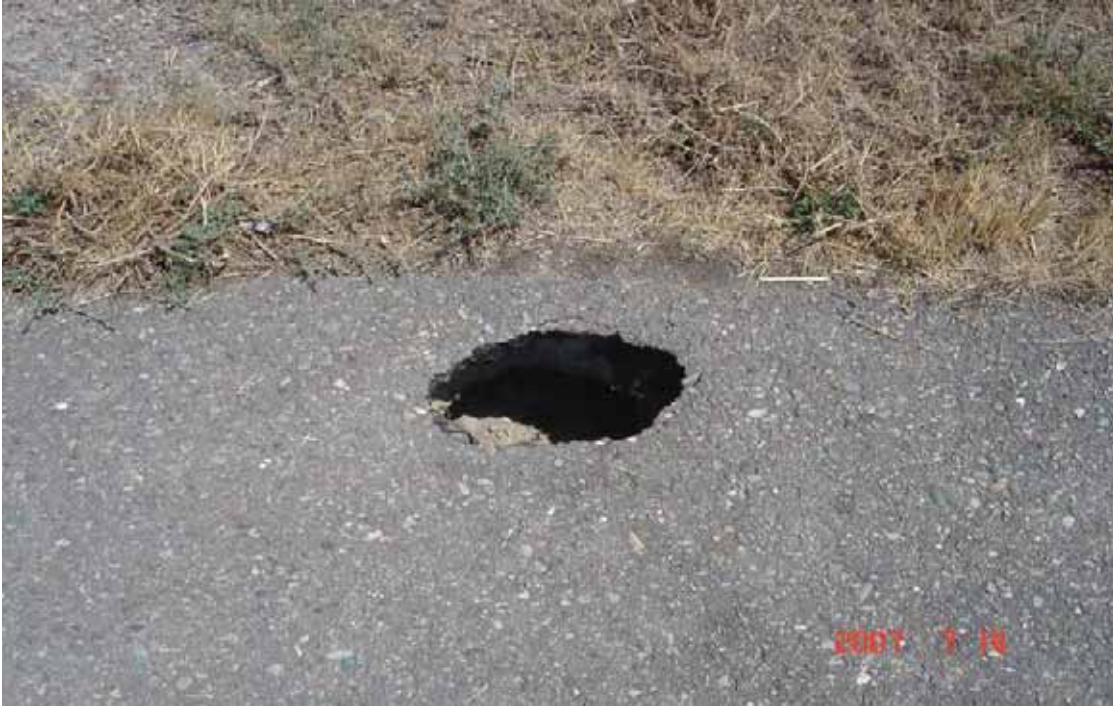
Photo # 6 - MP 0.16 - Erosion Deficiency
