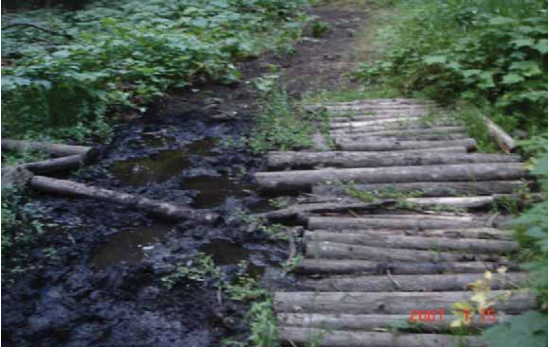
Photo # 13 - MP 1.29 - Drainage Deficiency, Puncheon
