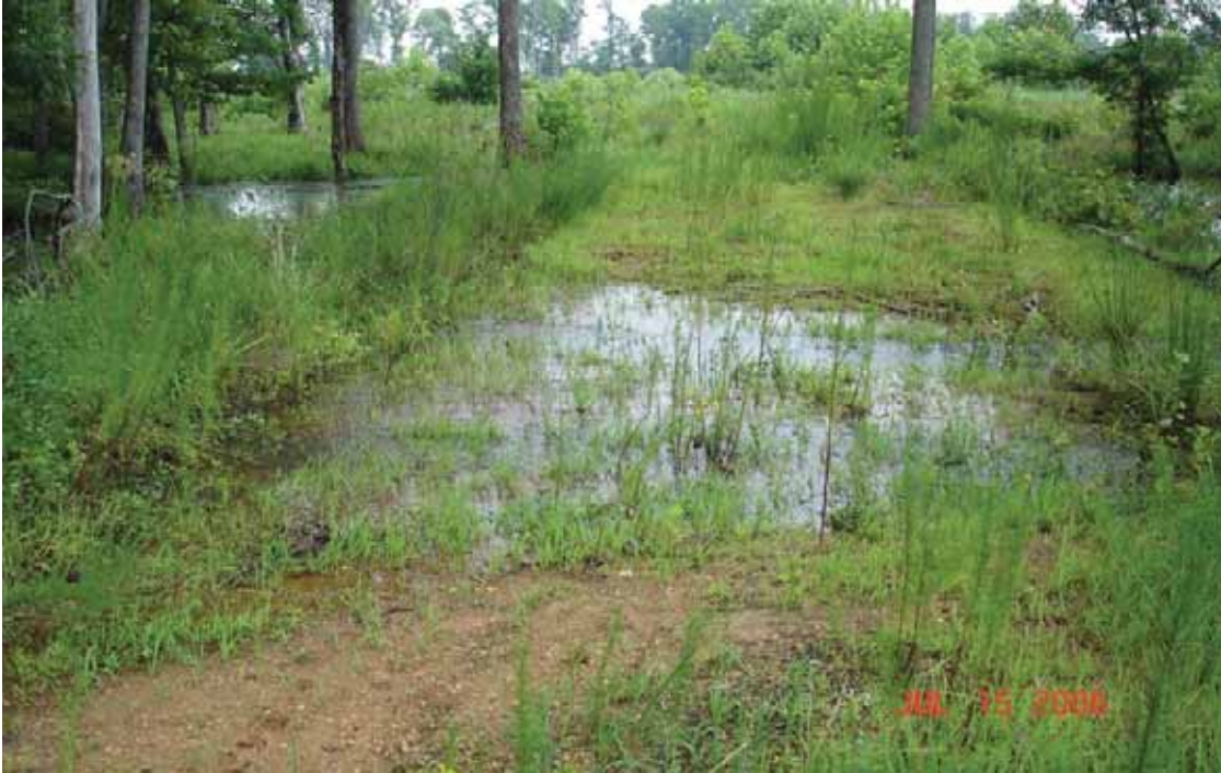
Photo # 7 - MP 0.44 - Drainage Deficiency
