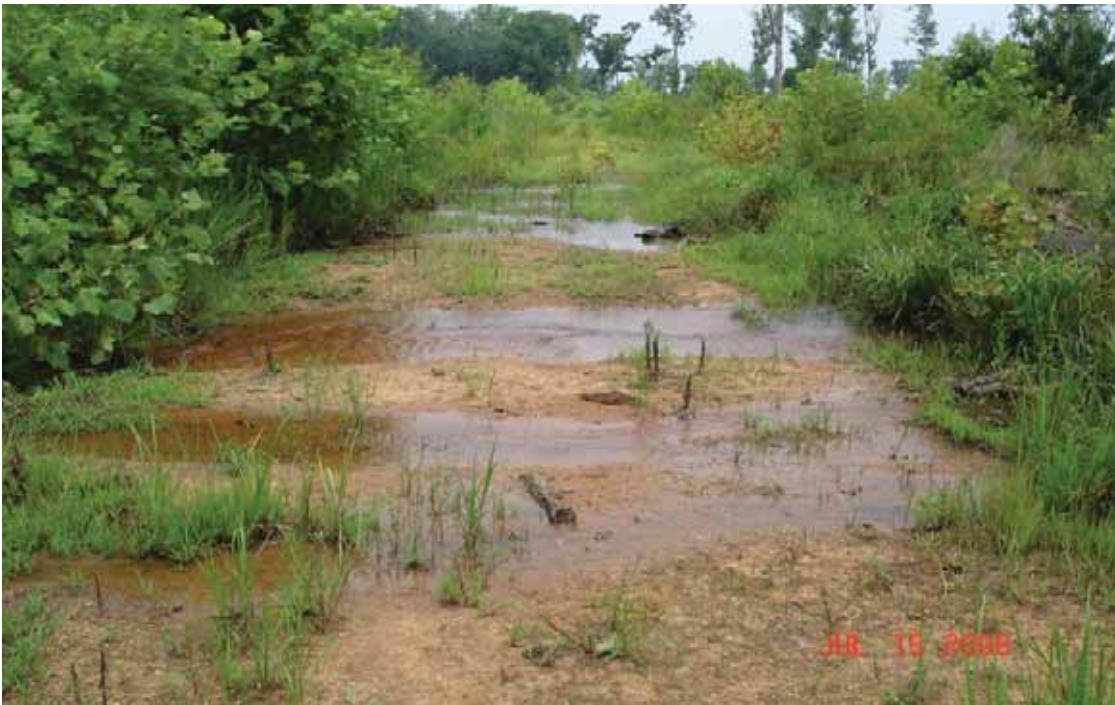
Photo # 6 - MP 0.61 - Drainage Deficiency
