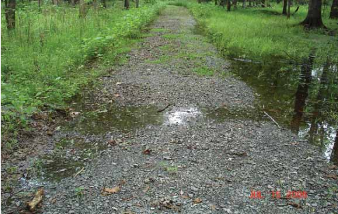
Photo # 16 - MP 0.63 - Drainage Deficiency
