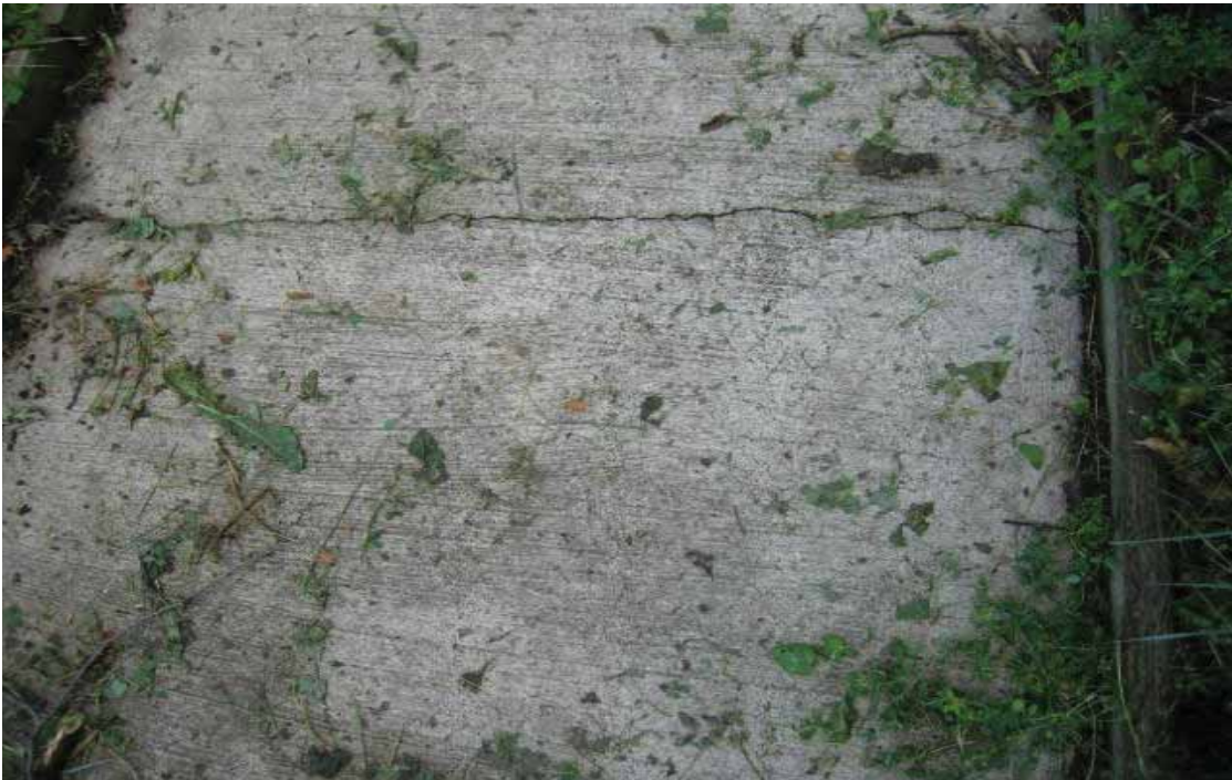
Photo # 2051 - MP 0.65 - Other Deficiency (Concrete cracking)
