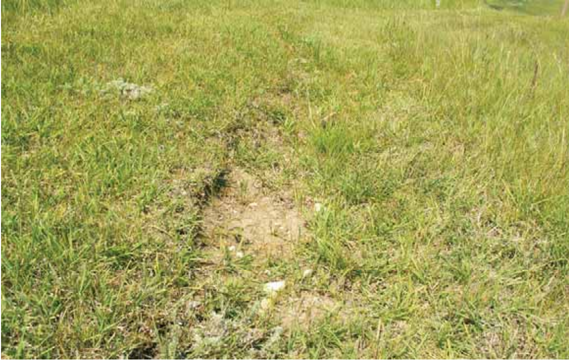
Photo # 160 - MP 0.22 - Other Deficiency (Slumped tread)
