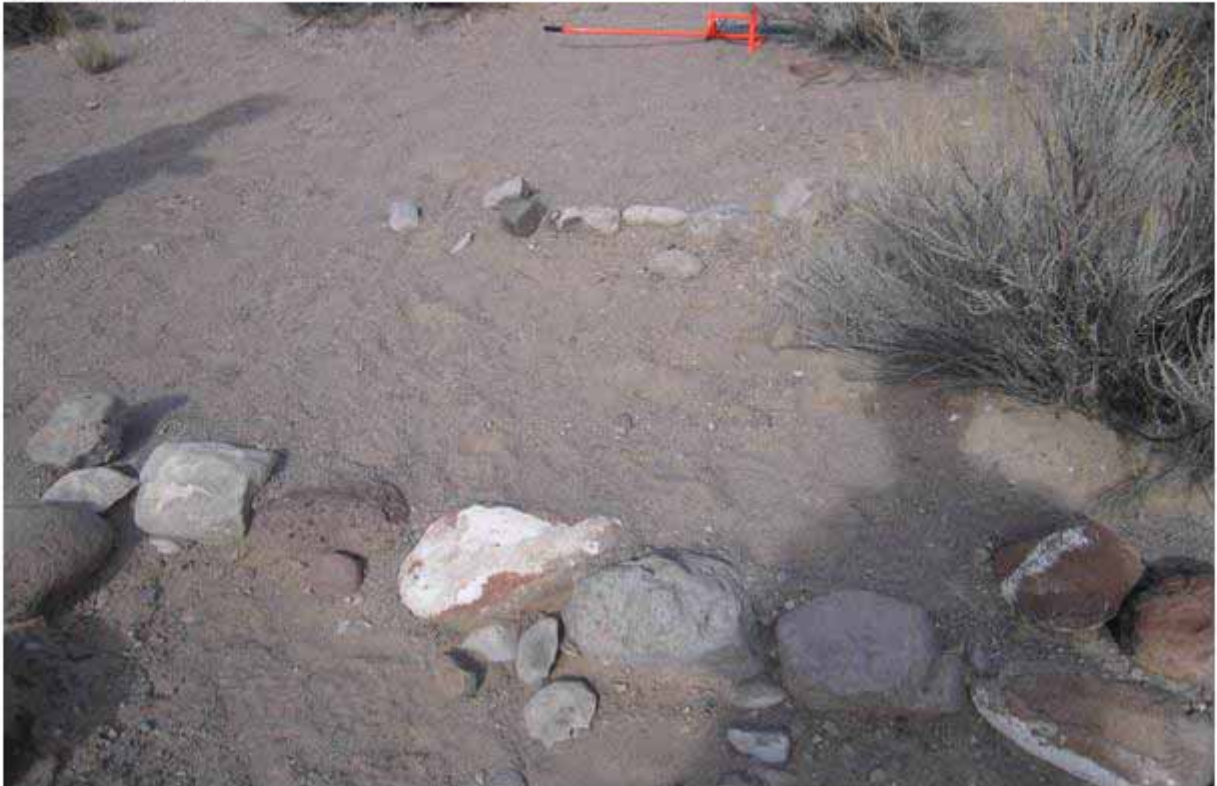
Photo #0459 - MP -Water Bar:Rock
